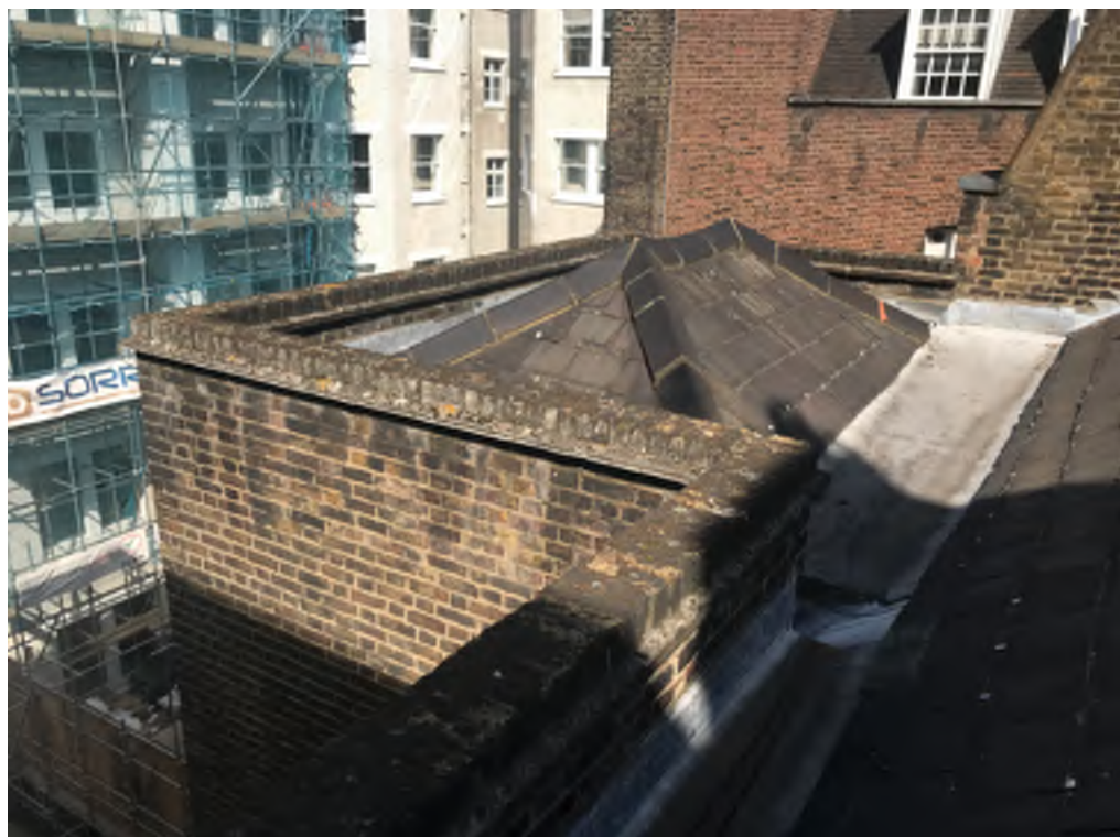
Photograph 6: Roof 5 view north west
