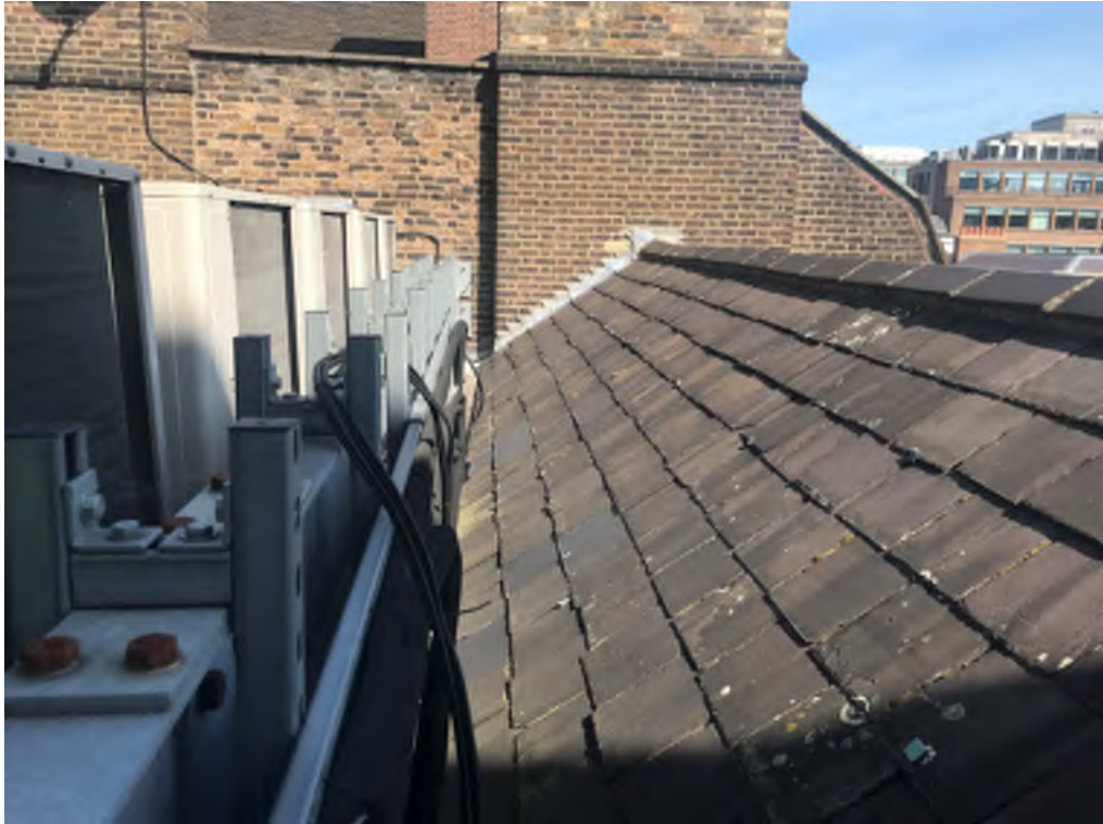
Photograph 3: Roof 1 view north
