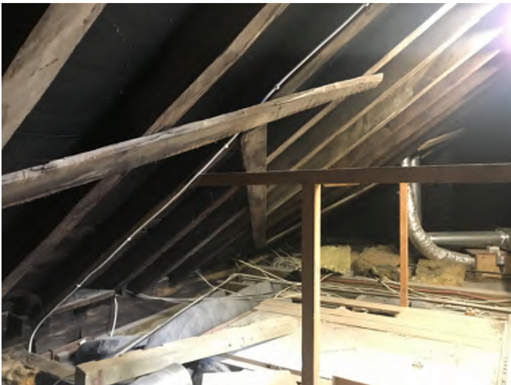
Photograph 14: Roof 3 view north west
