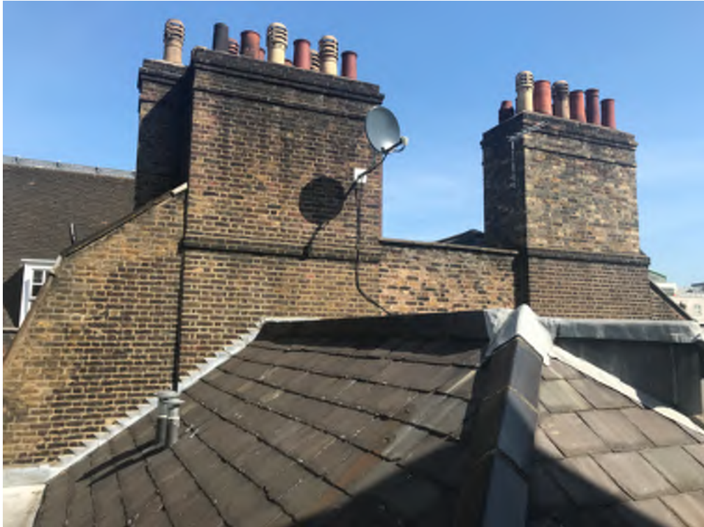
Photograph 25: North party wall showing sequential construction
