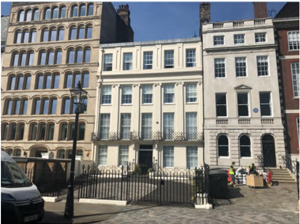
Photograph 2: Front elevation of No.64
