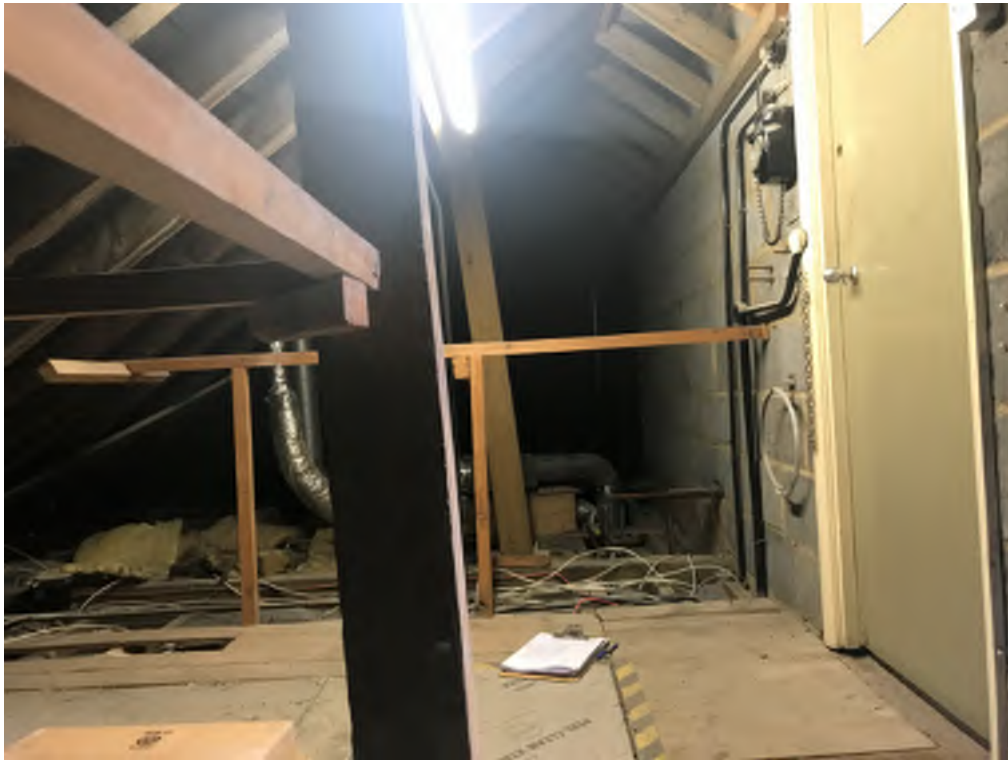
Photograph 13: Roof 3 view north
