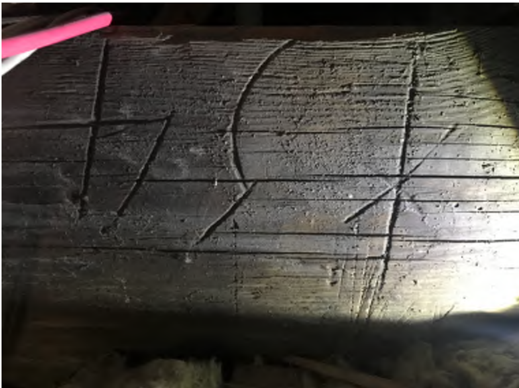
Photograph 22: Roof 3 primary beam detail showing shipping marks
