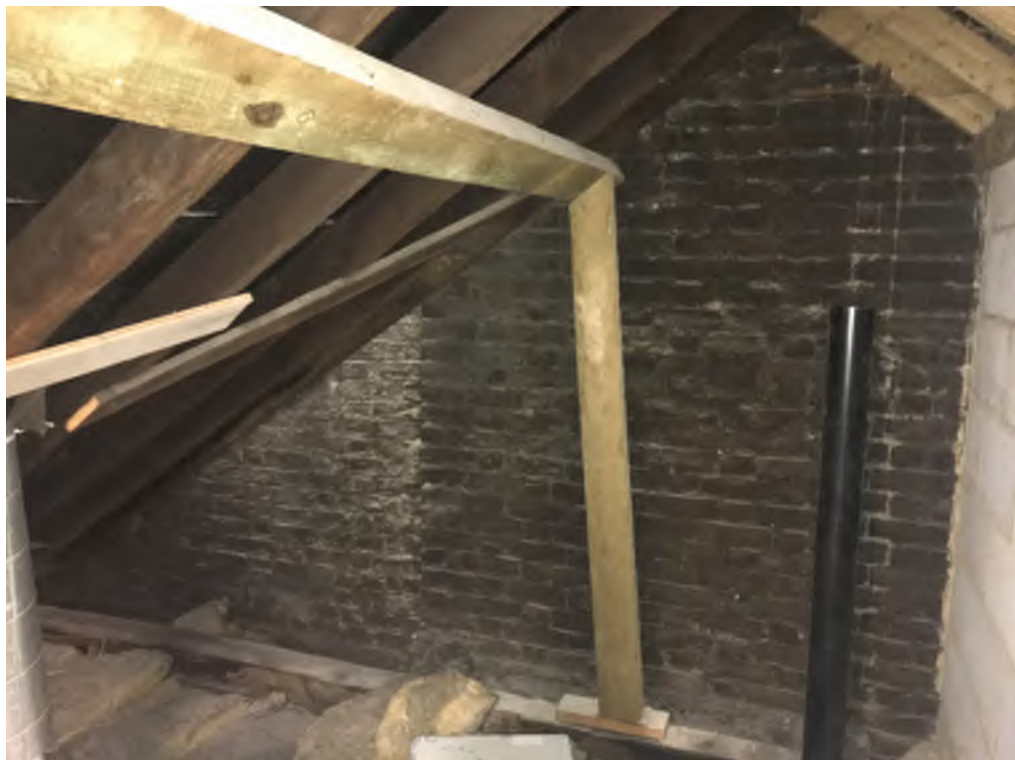
Photograph 28: Roof 3 north party wall showing previous duo-pitched roof profile
