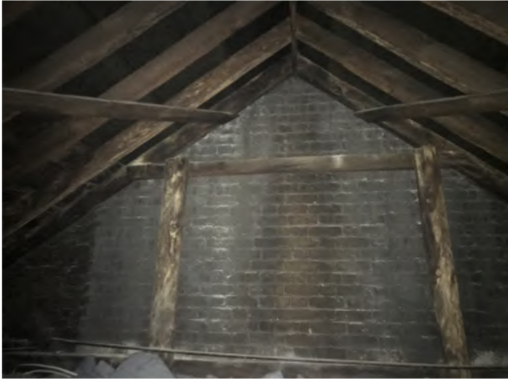
Photograph 27: Roof 1 north party wall with no evidence of previous roof profile
