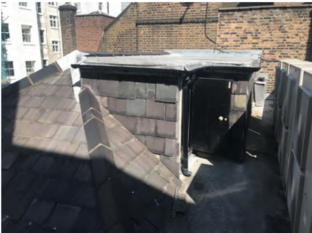
Photograph 4: Roofs 2 & 3 view north
