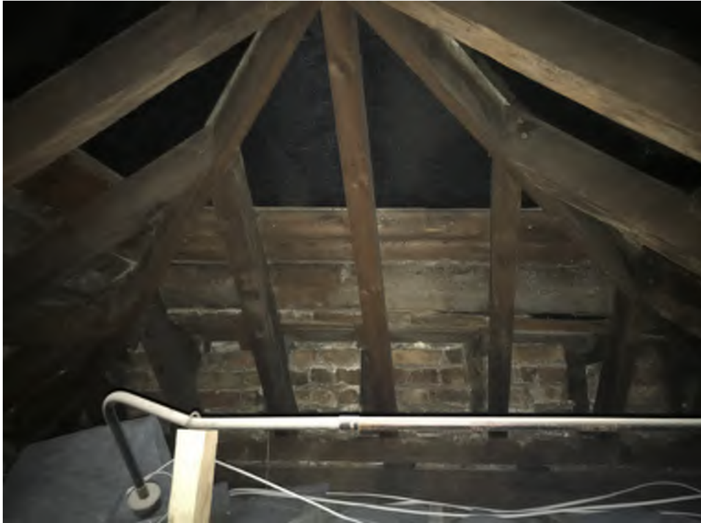
Photograph 23: Roof 5 view north
