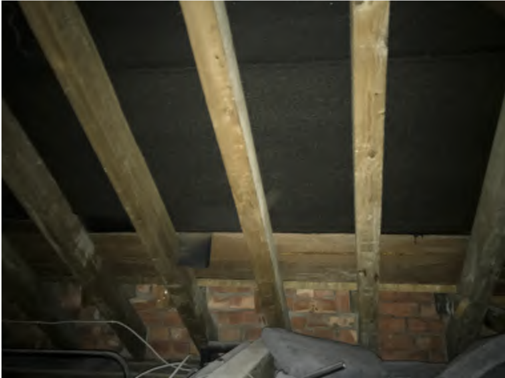
Photograph 9: Roof 1 view east
