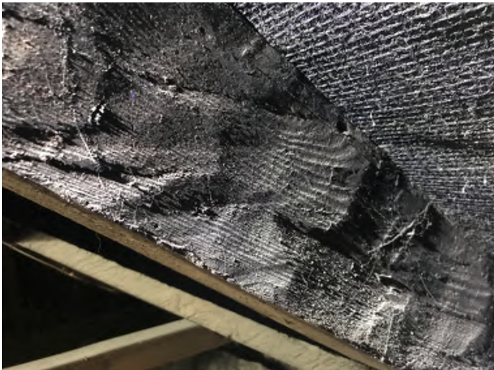
Photograph 18: Roof 3 rafter detail showing hand formed cutting marks
