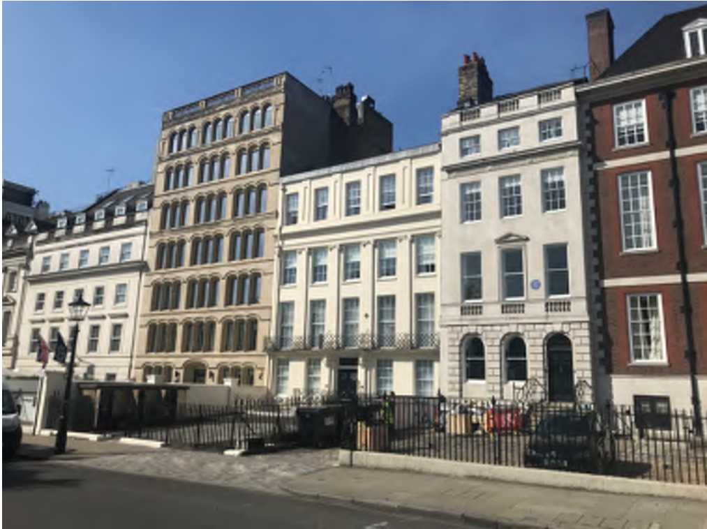
Photograph 1: Front elevation of No. 64 in context with adjacent buildings
