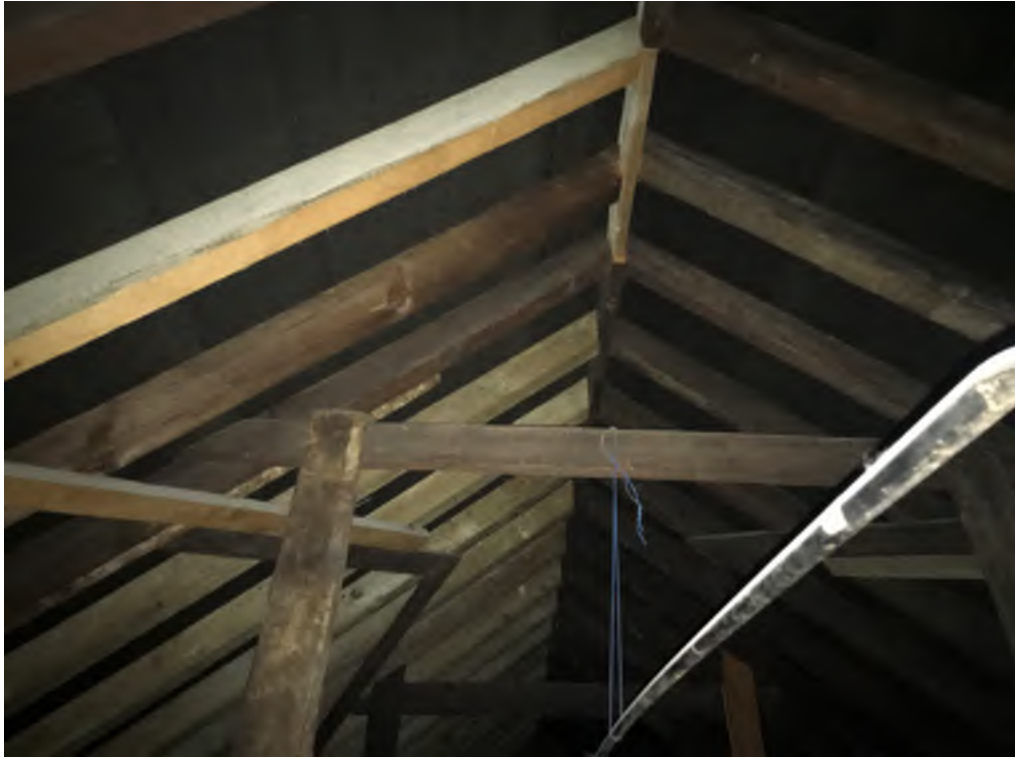
Photograph 7: Roof 1 view south
