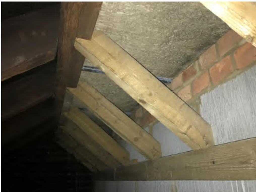
Photograph 12: Roof 2 view north
