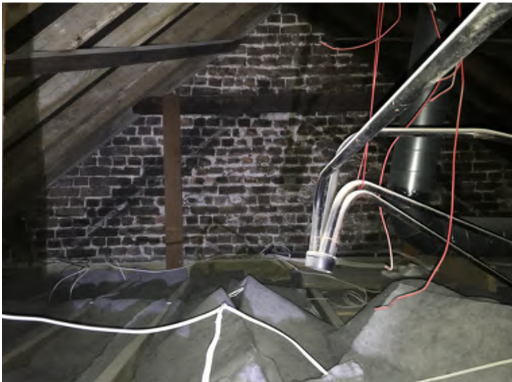
Photograph 26: Roof 1 south party wall showing previous duo-pitched roof profile
