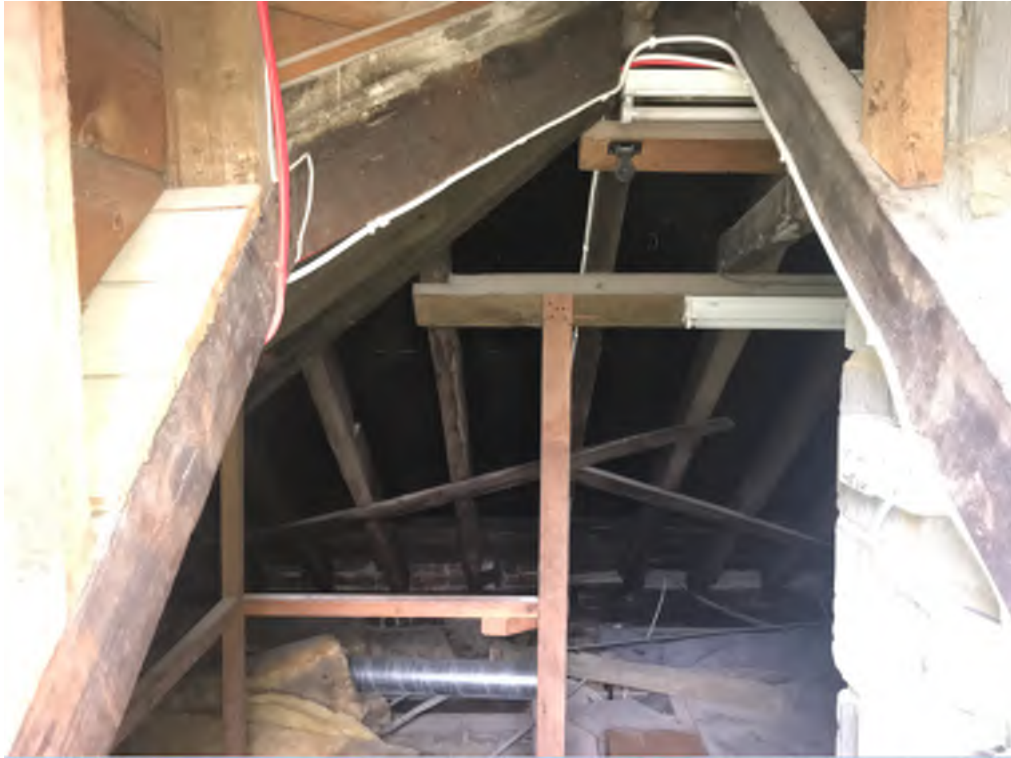
Photograph 15: Roof 3 view west
