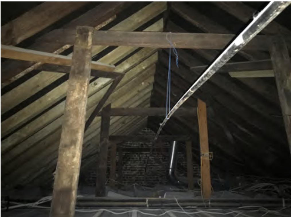
Photograph 8: Roof 1 view south
