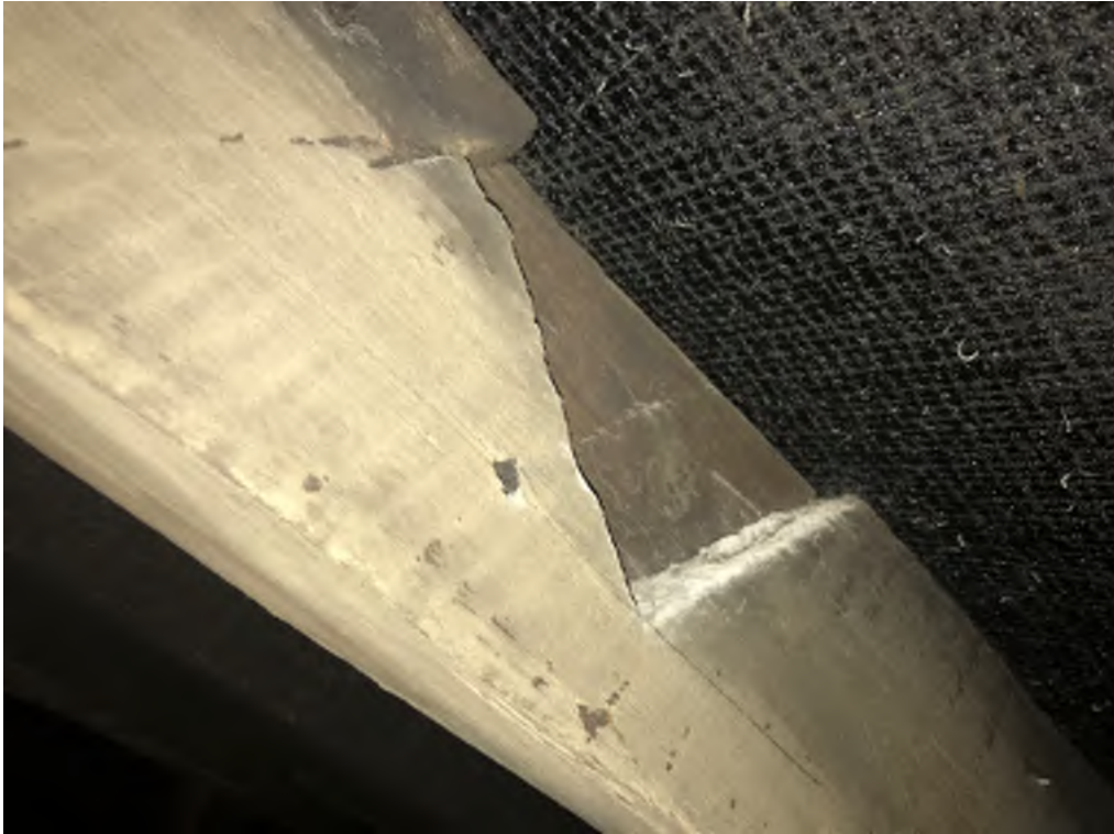
Photograph 19: Roof 3 rafter detail showing reused common rafter
