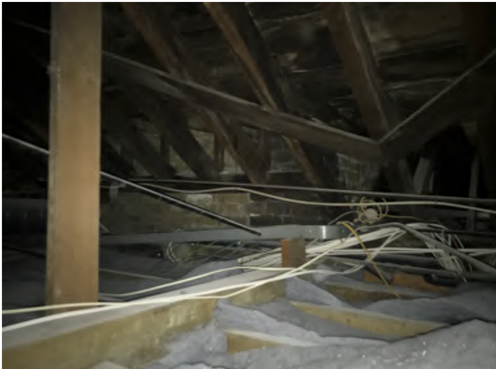
Photograph 10: Roof 1 view south west
