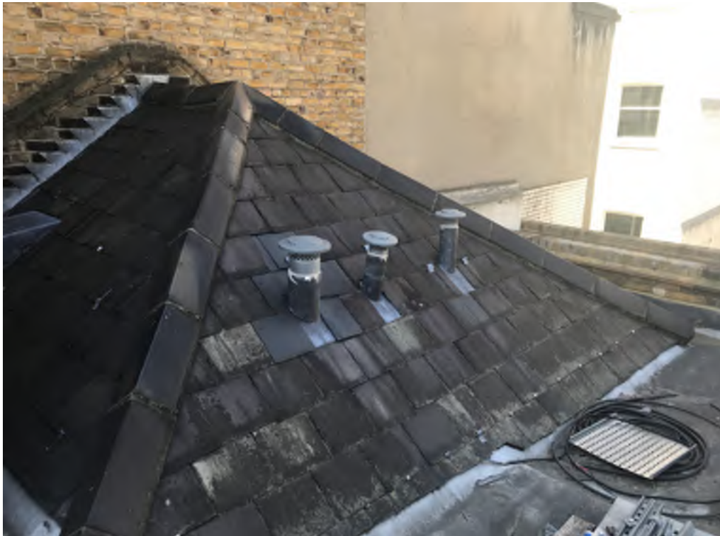
Photograph 5: Roof 4 view south west
