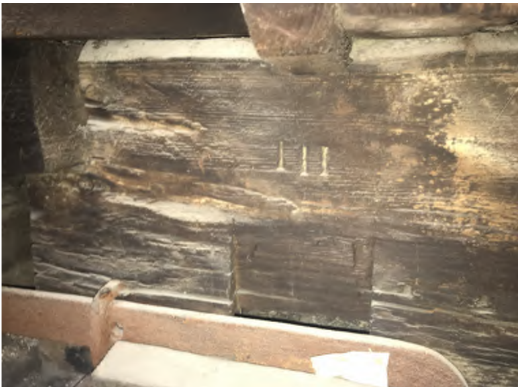
Photograph 20: Roof 3 primary beam detail showing carpenters' assembly mark
