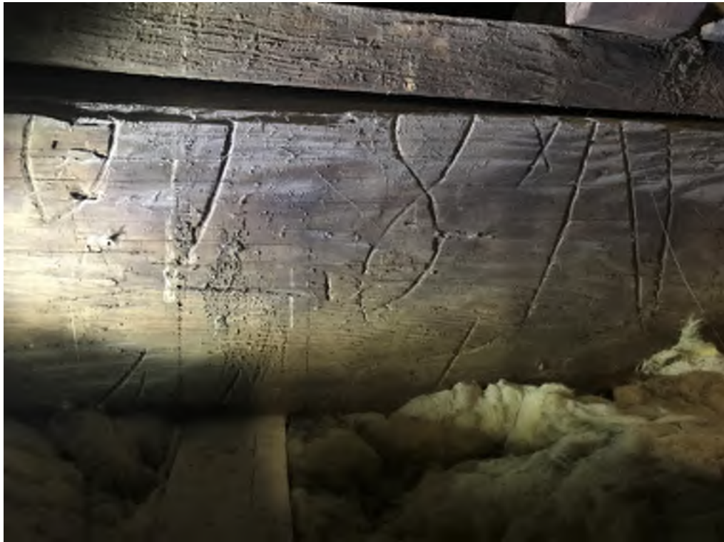
Photograph 21: Roof 3 primary beam detail showing shipping marks
