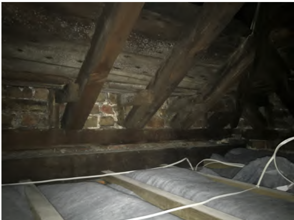
Photograph 24: Roof 5 view west
