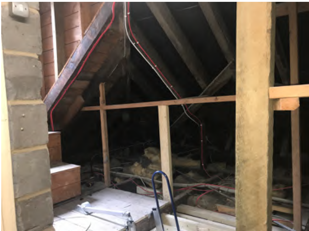
Photograph 16: Roof 3 view south east
