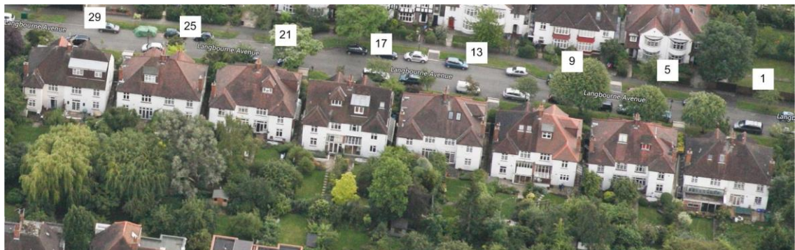
Rear of Langbourne Avenue houses, north side (odd nos)
