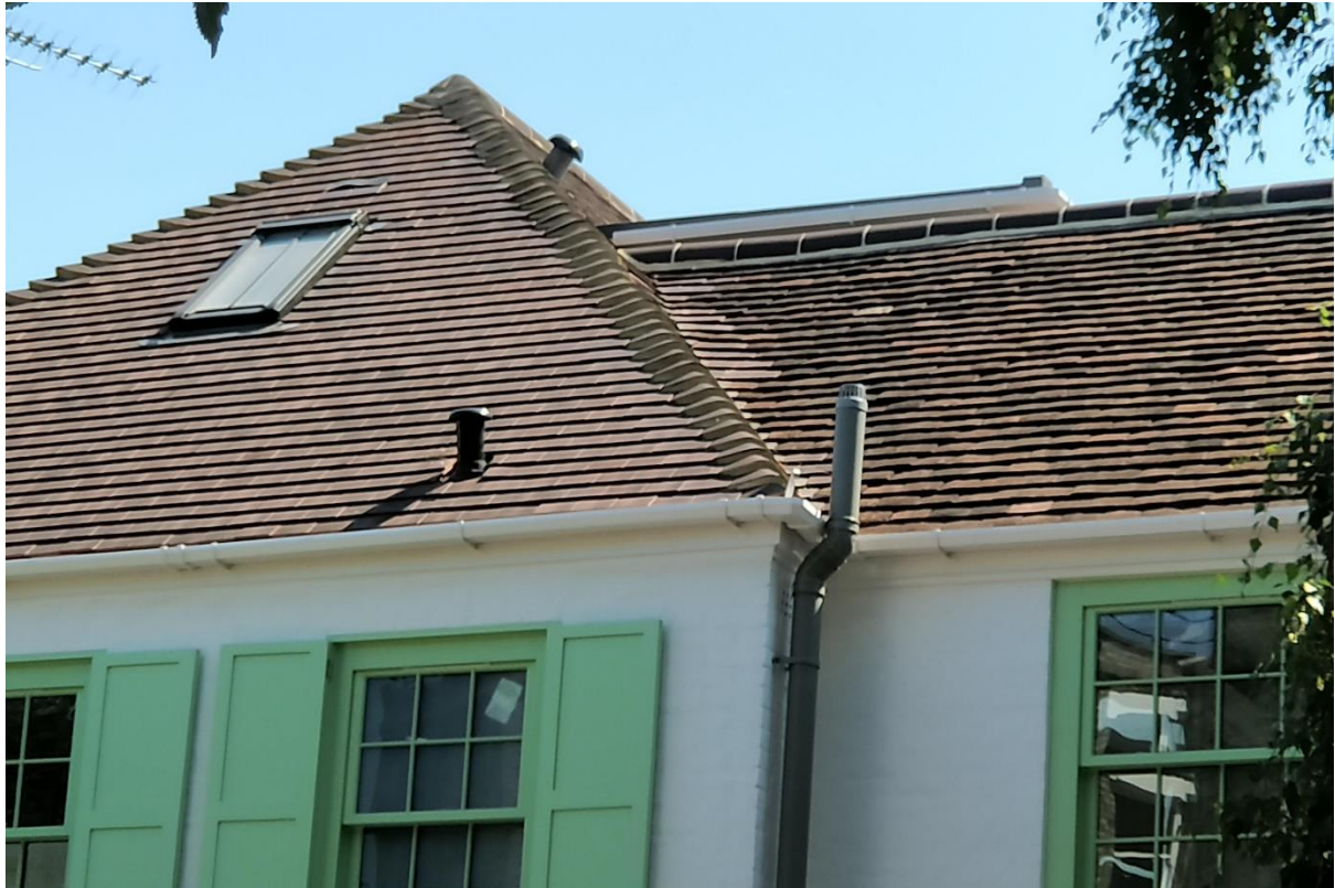
Example of openable roof window and roof natural ventilation – 42 Pilgrim’s Lane
