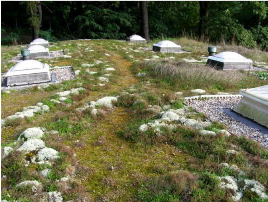
Established Sandy Heath Roof System (>5 years) Teufelssee, Berlin-Gruenwald (Germany)
