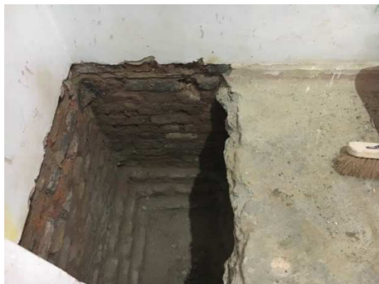
Photo 3: Lower ground floor trial pit
