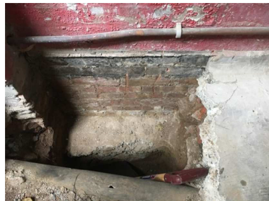
Photo 4: Ground floor trial pit in 1960s extension
