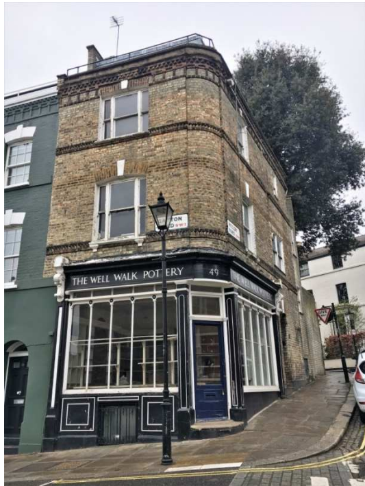
Photo 1: Gayton Road (East) Elevation
