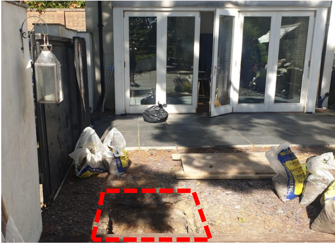
Figure 3: Trial Pit Location
