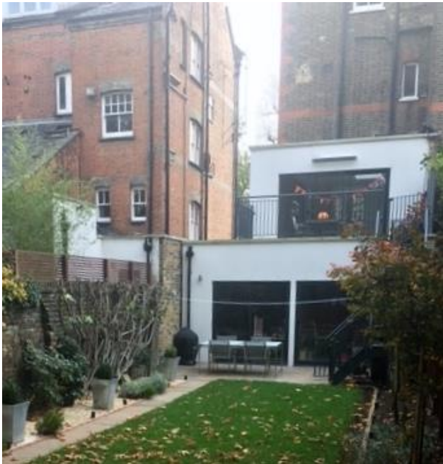
View of extension site from the garden of 100 Fellows Road
