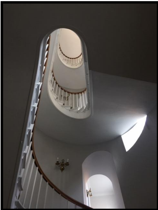
Figure 8 Existing Internal Staircase
