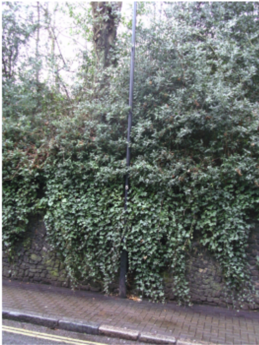
LOCATION A (LAMP POST)
