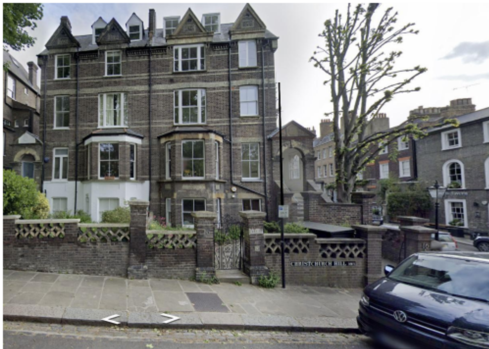
LOCATION A WITH POLE
