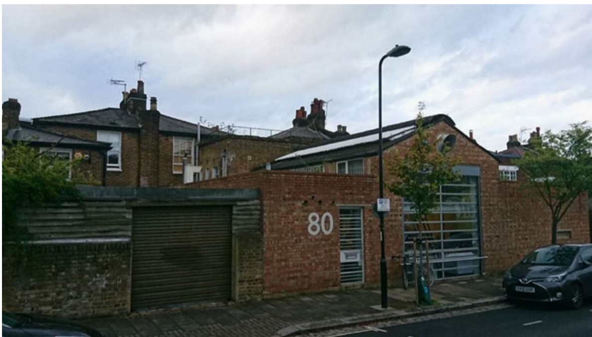
Fig 4: Street front view from west
