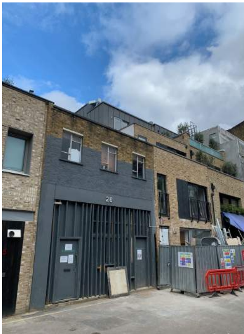
Works in progress at the site
