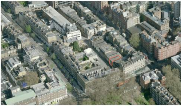
Fig 2. Bird's eye view Looking North - site marked in red
