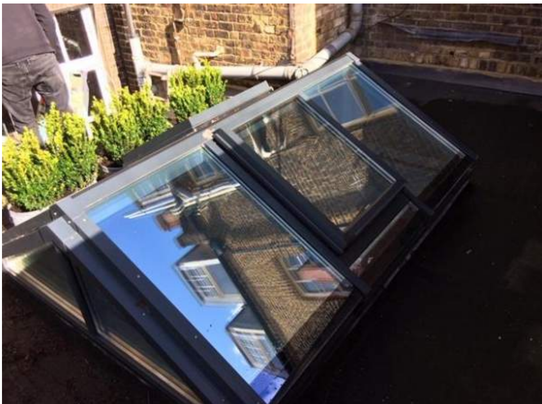
5. Rooflight with reflective glazing
