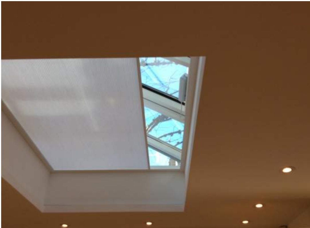
5. Rooflight with reflective glazing
