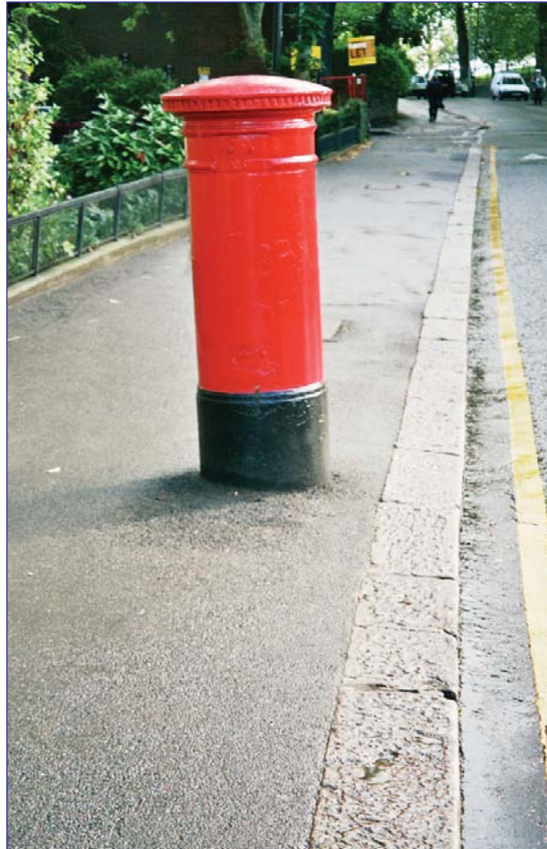
New bituminous footway on Regent's Park Road
