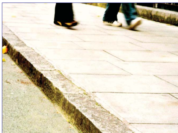
Boulevard paving laid with 150mm staggered bond
