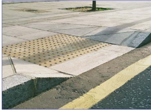
Details of dropped kerbing in John St
