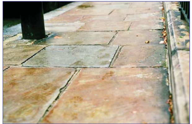
Old York stone re-laid with flush pointing
