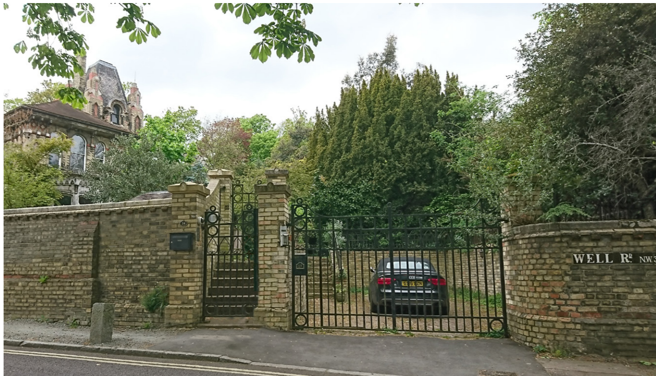
FIG. 14. EXISTING NO.18 (LEFT) AND NO.17 (RIGHT) ACCESS GATES TO BE RETAINED
