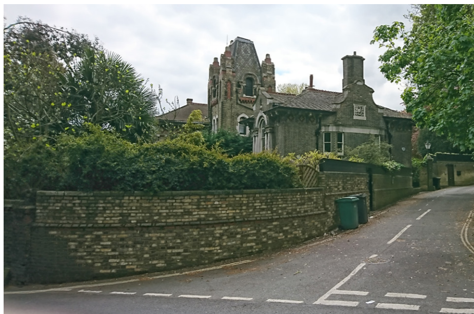
FIG. 07. VIEW 1: EXISTING BOUNDARY WALL TO NO.1 CANNON LANE FROM EAST HEATH ROAD
