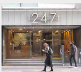
Lack of level access.
