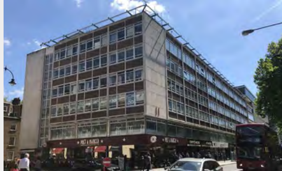
Existing building: 247 Tottenham Court Road
