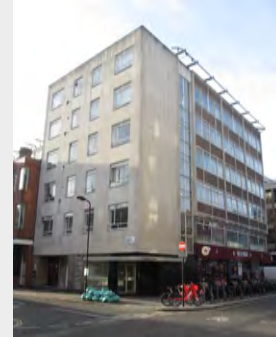
Existing building: 3 Bayley Street
