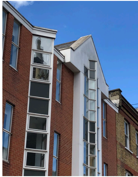
Photograph 4.2: Exterior of B1 (4 Morwell Street), eastern aspect
