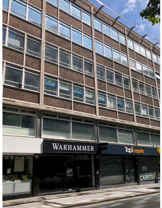
Photograph 4.10: Exterior of B5 (247 Tottenham Court Road), western aspect
