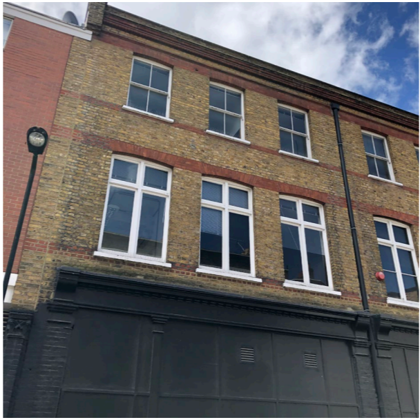
Photograph 4.3: Exterior of B2 (2 Morwell Street), eastern aspect
