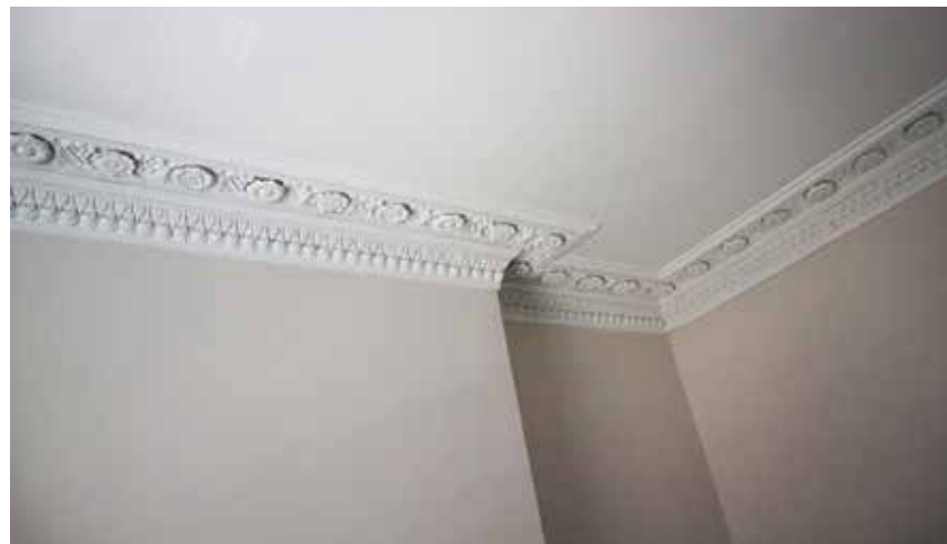
3.10 Detail of cornice and plasterwork in first floor front room (Insall, 2019)
