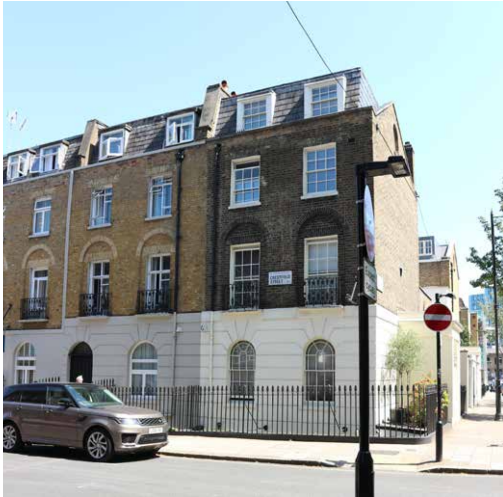
3.3. Front elevation of 1 Crestfield Street (Insall, 2019)
