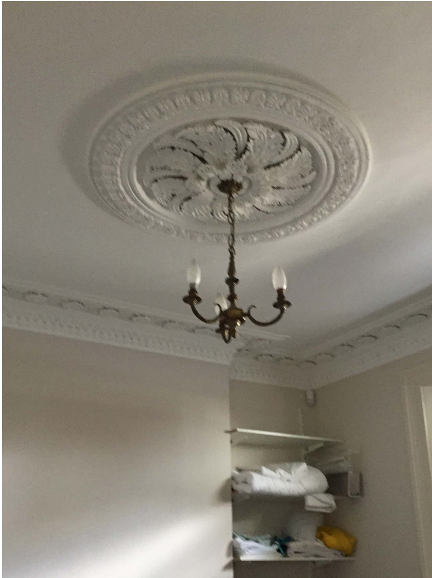
Fig 3. First Floor Bedroom 2, existing ceiling rose
