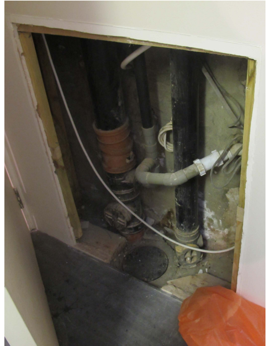
Fig 8. Basement utility room, view within access hatch (access hatch visible within Fig 7) showing boxing out, hidden services and contentious tanking system.
