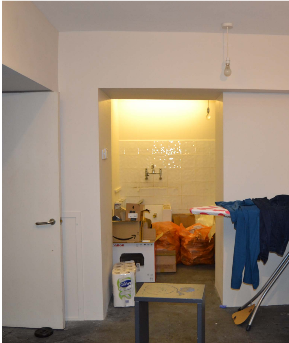
Fig 7. Basement utility room, view of rear wall of building above with modern plasterboard boxed out to conceal services and tanking systems.
