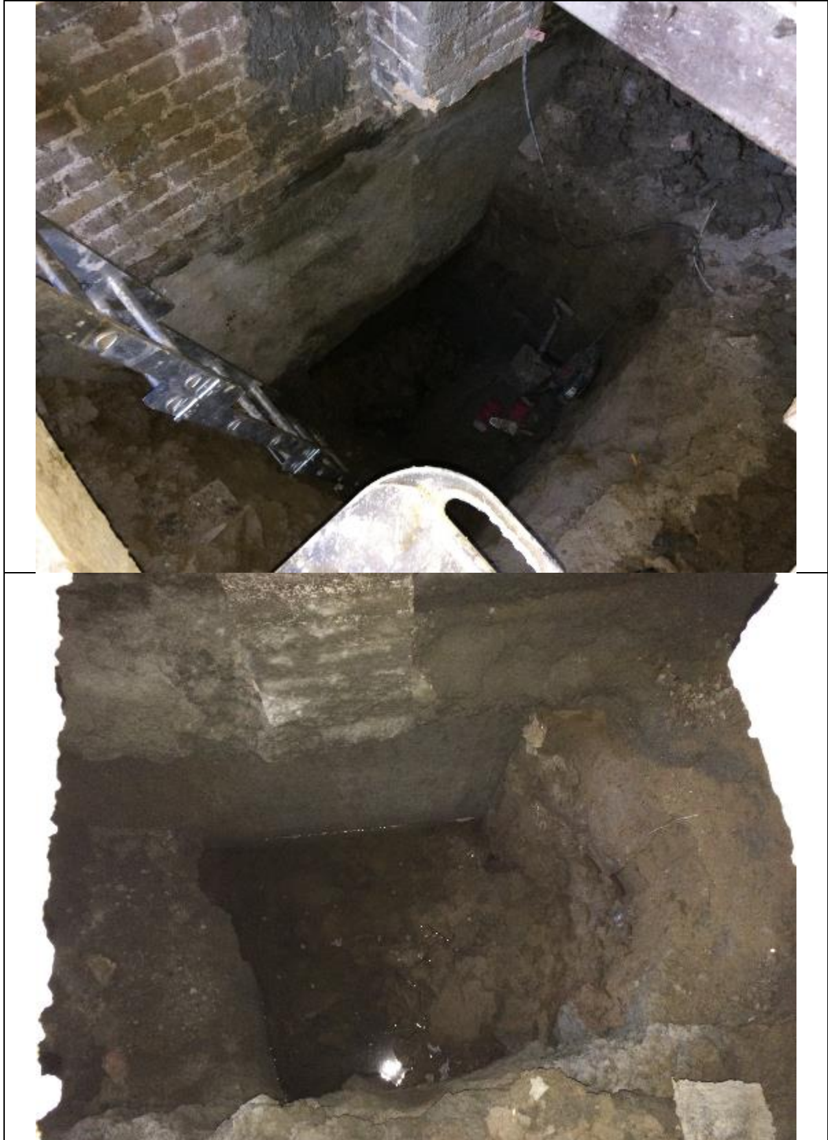
2016-11-16 The excavation starts for the East Side underpinning
