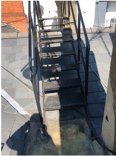
Escape stair over roof
