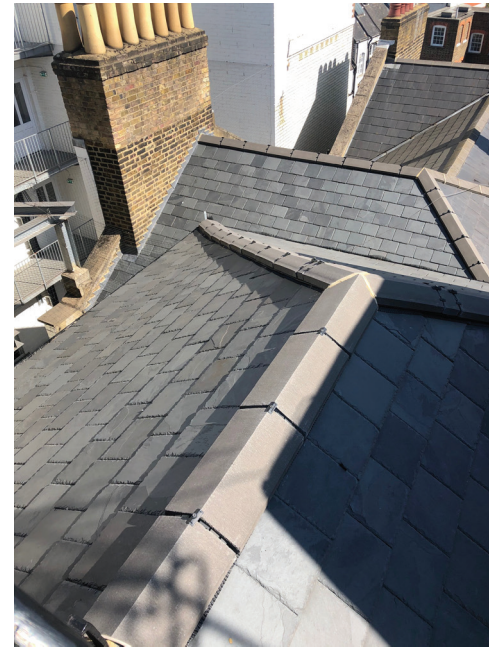
Roof of bedroom looking northeast
