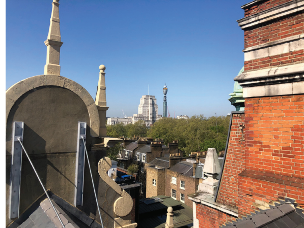
Rear of decorative gable on front facade
