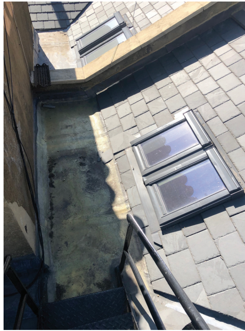
Existing escape route and skylights
