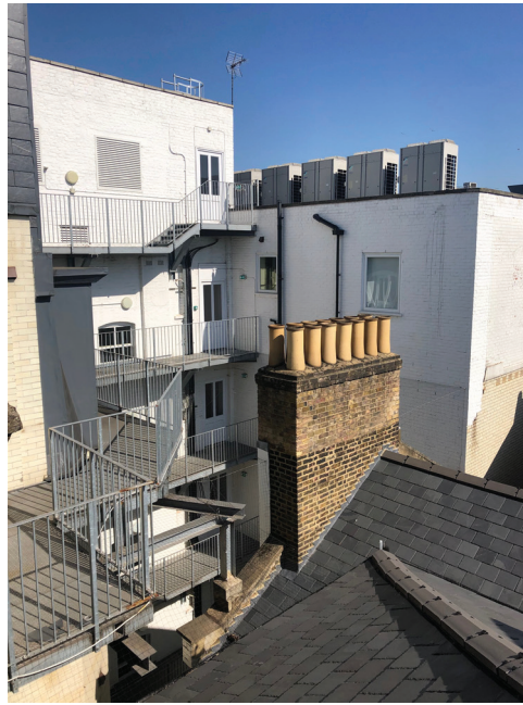
Roof of bedroom looking north
