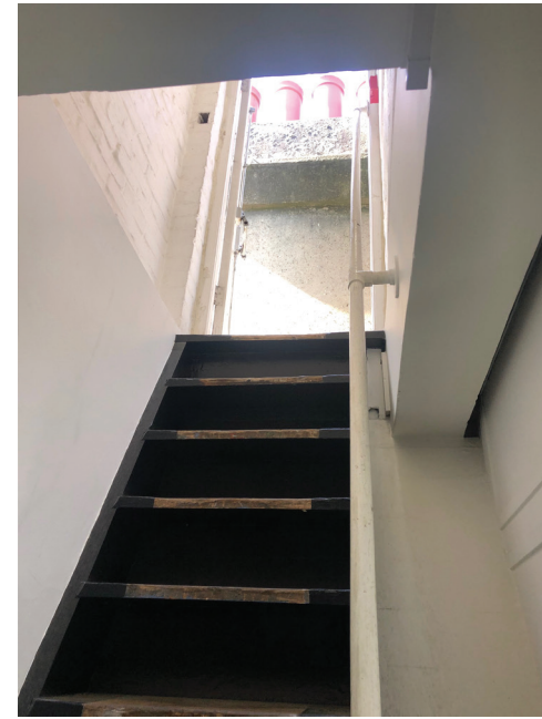
Roof access stair looking up from 6th floor
