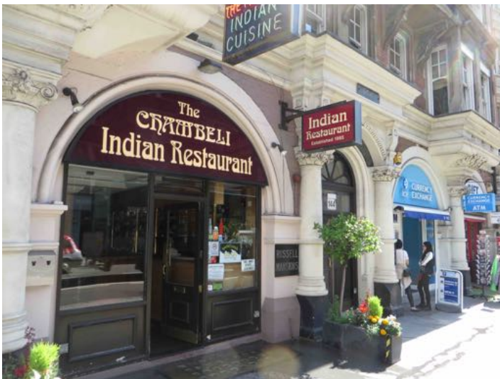
Arched shopfronts, stone main entrance portico, decorative capitals
