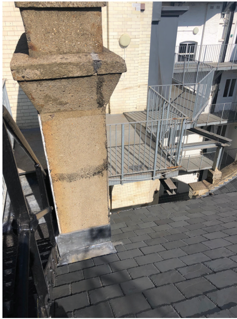
Roof of bedroom looking northwest
