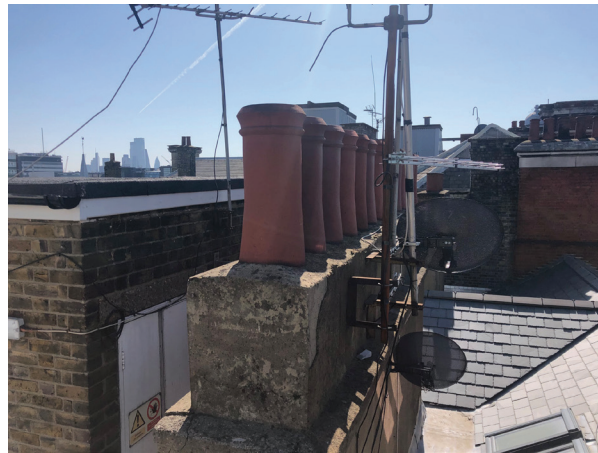
Chimneys and stairwell building on 7th floor
