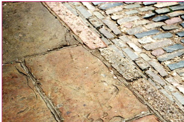
York stone and old granite setts
