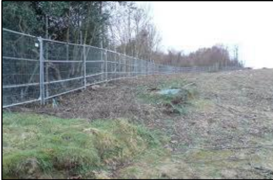
Tree protective fencing example.
