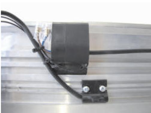
Place the second release component at about 300mm from the centre of the electric lock and fasten it with two self-threading screws supplied in the Kit.
