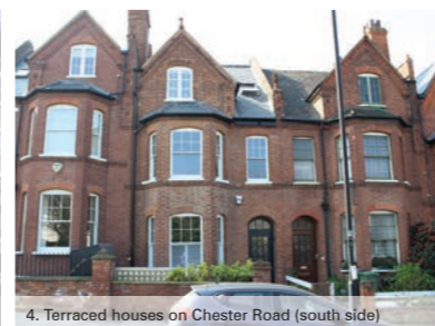
4. Terraced houses on Chester Road (south side)
