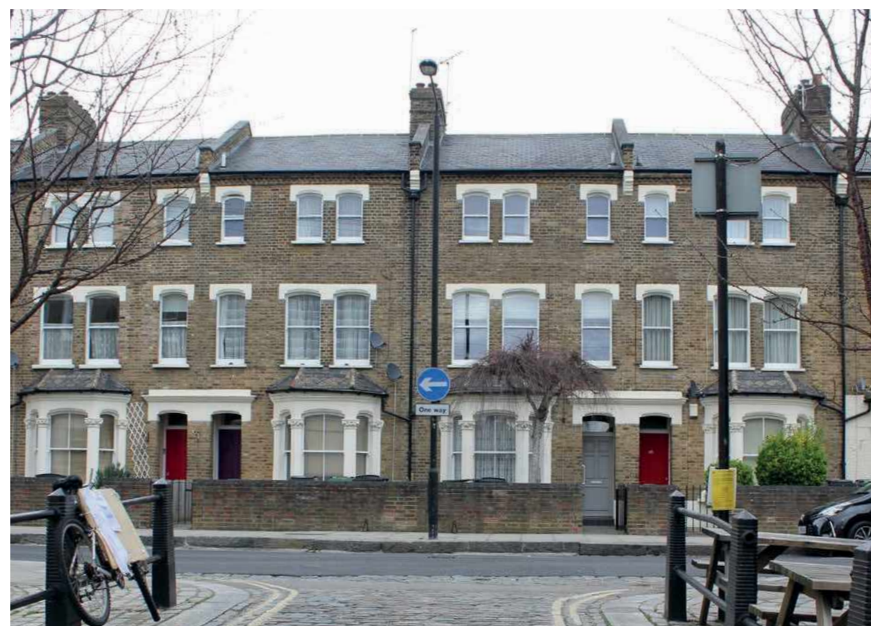
Terraced houses that make a positive contribution to the Conservation Area, adjacent to the site along Chester Road.
