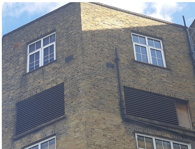
Photograph 3: The second new damaged ventilation feature recorded at a height of 9m on the north east face of the Victoria Wing of building B1 during the PRA.
