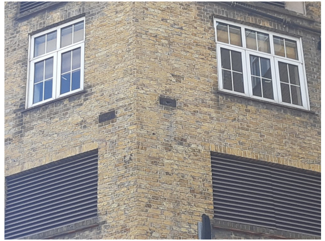
Photograph 2: The first new damaged ventilation feature recorded at a height of 6m on the north east face of the Victoria Wing of building B1 during the PRA.
