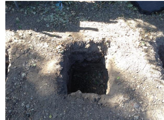
Fig 5 – Sample excavations for similar projects where careful hand digging is used and footing locations manipulated to reflect the presence of any root >25mm in diameter.
