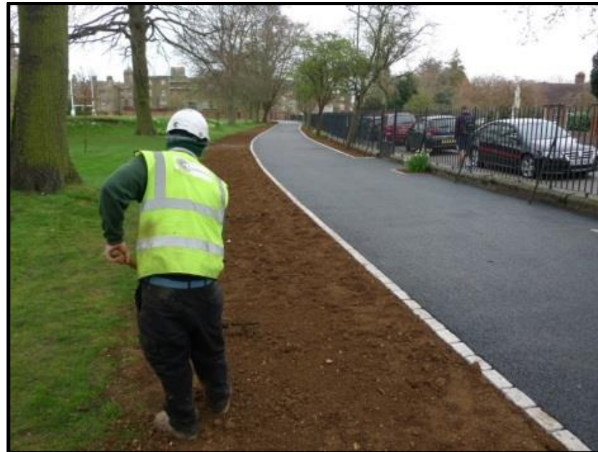
Fig 8 – In the event of 'making good' topsoil will be BS3882 compliant and raked out by hand to no greater depth than 100mm
