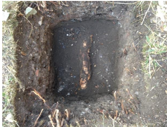
Fig 5 – Sample excavations for similar projects where careful hand digging is used and footing locations manipulated to reflect the presence of any root >25mm in diameter.
