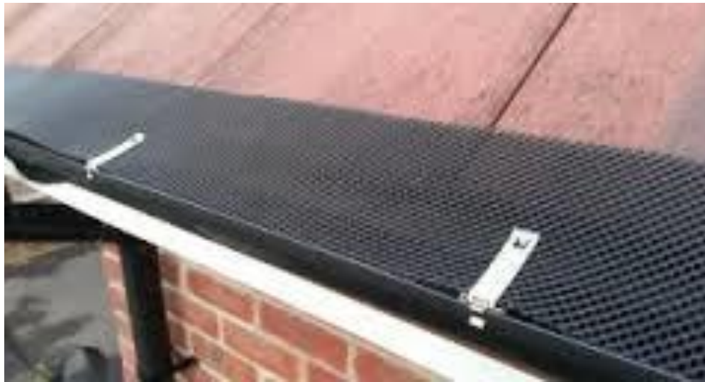
Fig 8 - Suitable gutter guards (2 types shown above) should be fitted to ensure that leaf drop from adjacent trees does not block new guttering leading to potential pressure for tree works.
