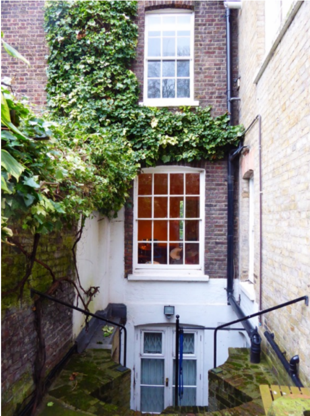
5) Rear elevation of adjoining no.7 (boundary wall to the left)
