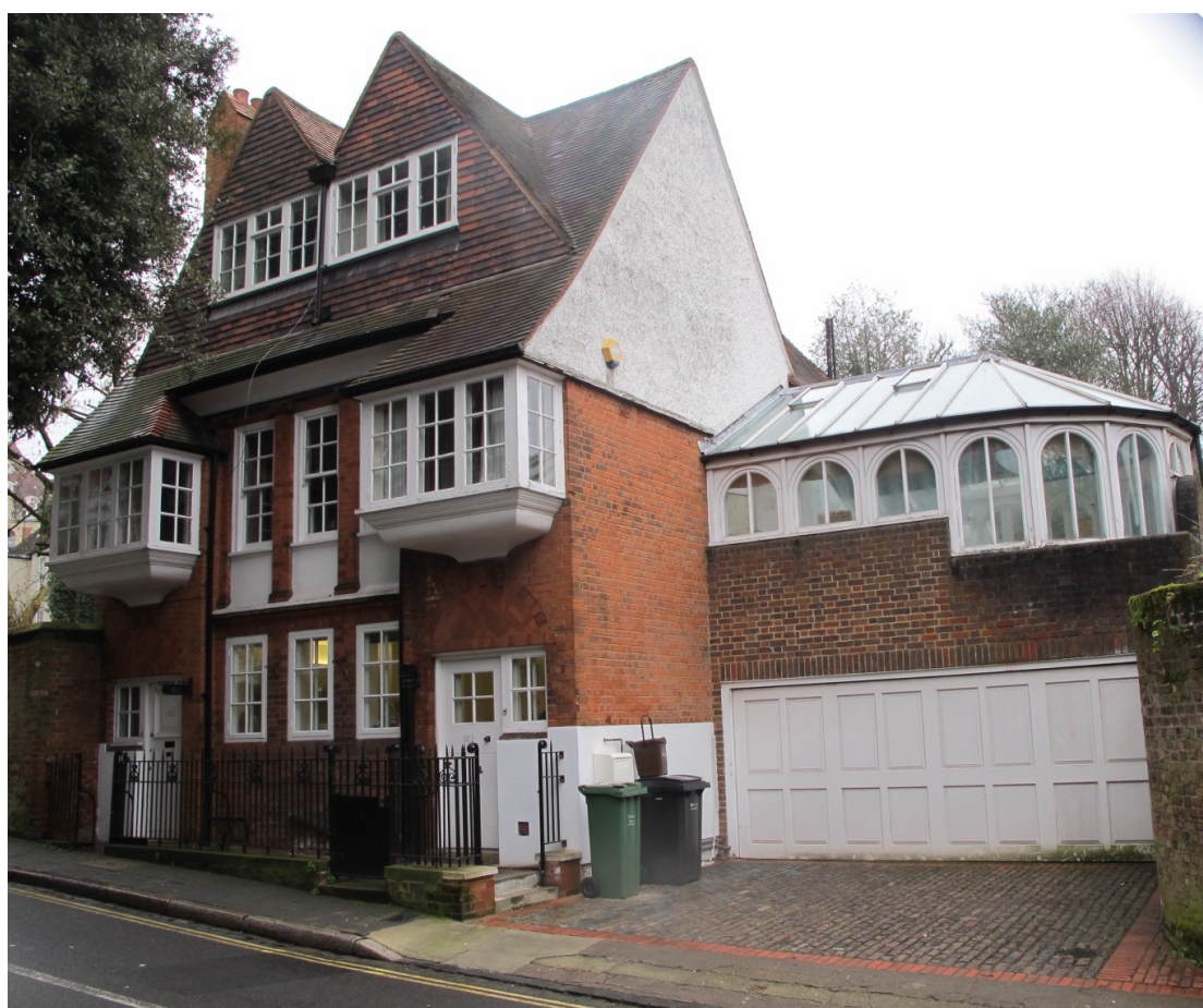
Image 01: View of 102 Frognal June 2020 from the street showing existing garage and conservatory
