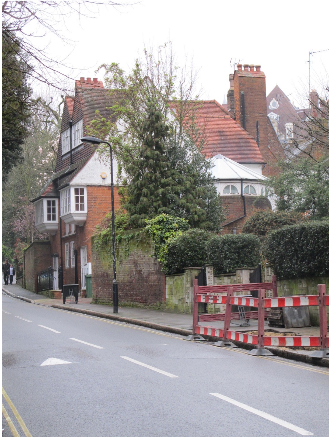
Image 03 View of 102 Frognal from south March 2020 showing current conservatory over garage and characteristic high brick garden wall
