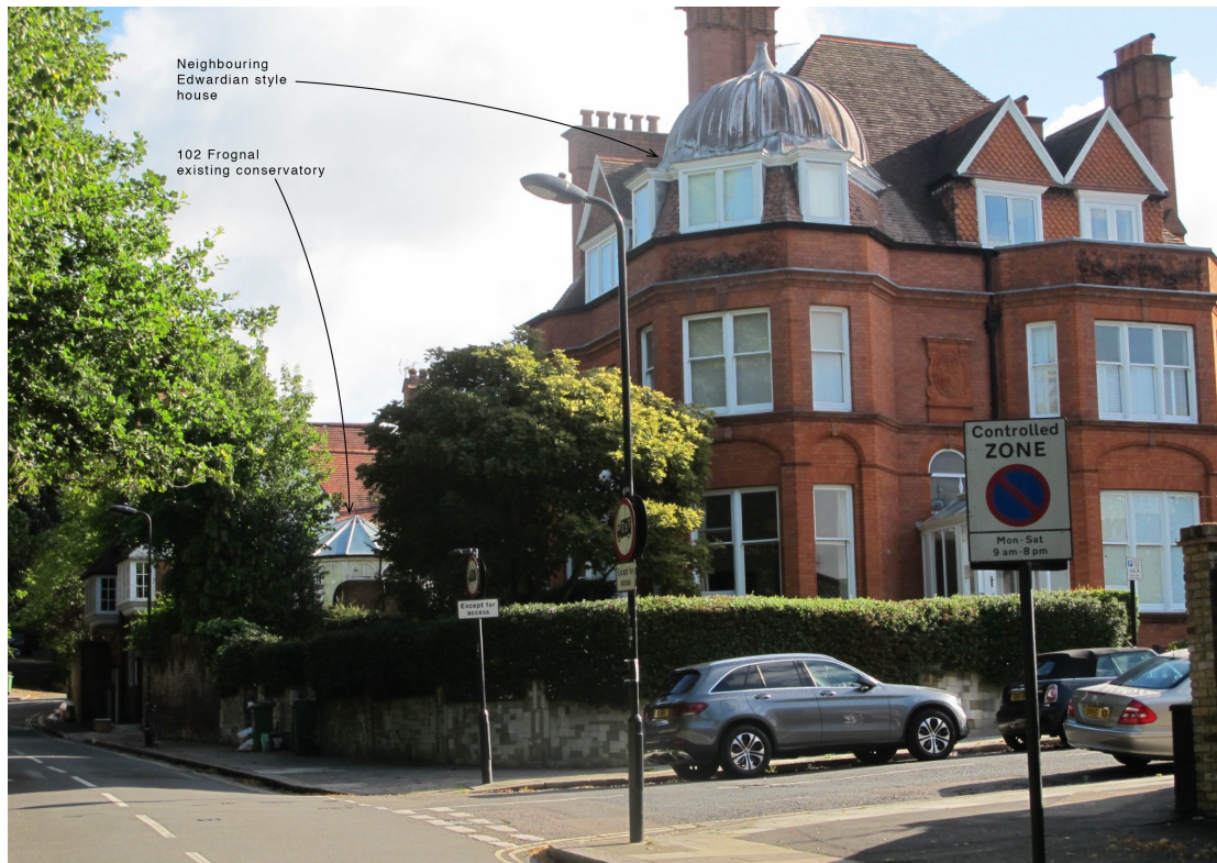
Image 02: View June 2020 taken looking north along Frogna1 towards 102 showing context within Hampstead Conservation Area
