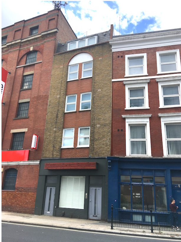
4.2 The property viewed from York Way with 5 & 6 storey neighbouring buildings
