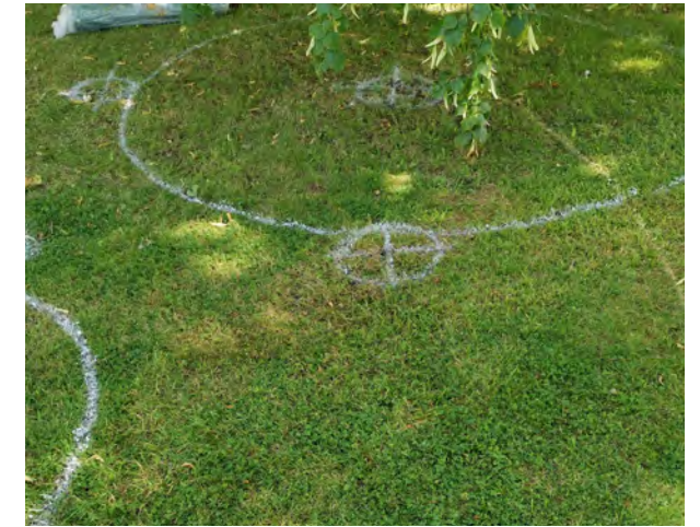
B. Setting out ground screw locations
