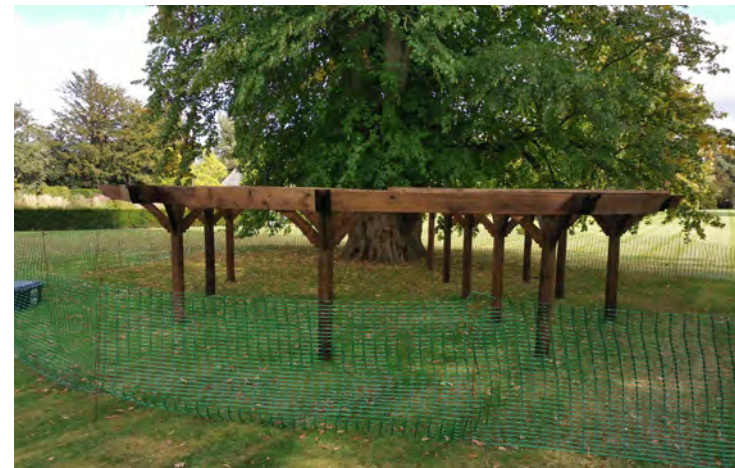
C. Erection of Playhouse platform
