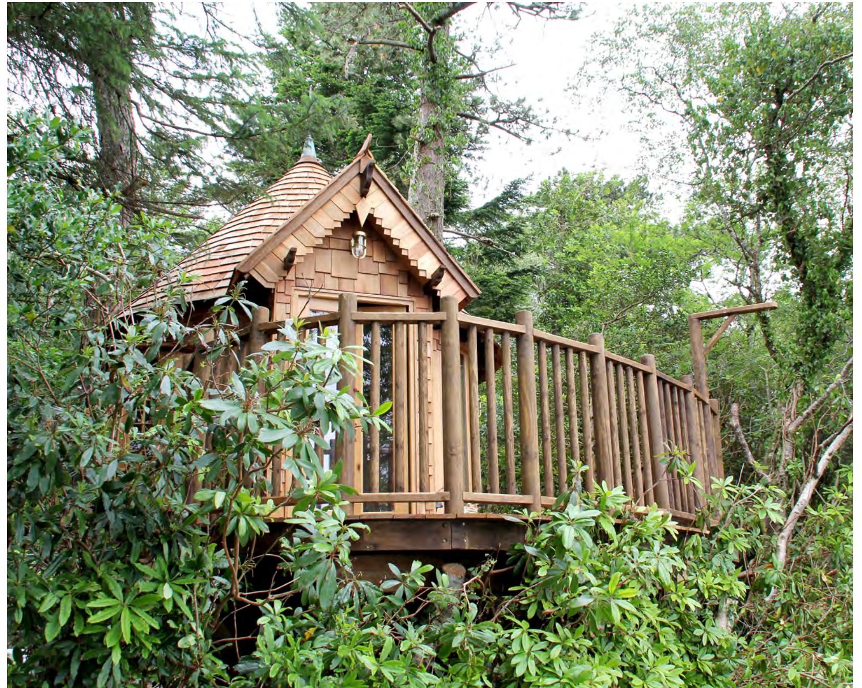
Image 1 : Precedent image showing similar playhouse supported using solid posts with elevated deck platform (N.B. not actual playhouse)
