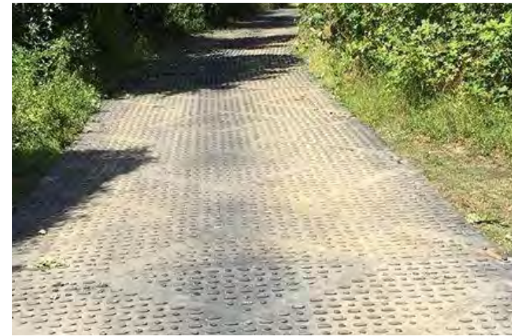
A. Temporary ground protection (if wet)
