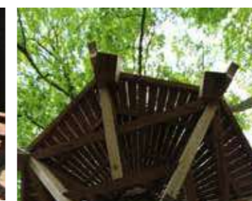
7. Softwood Substructure
