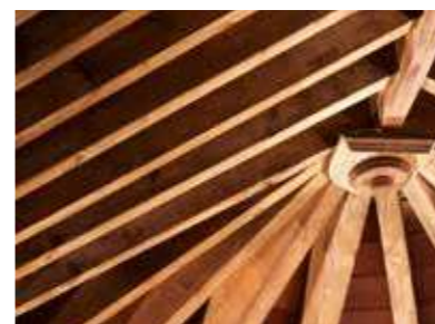
2. Soft Wood Rafters With Cedar Sarking Boards
