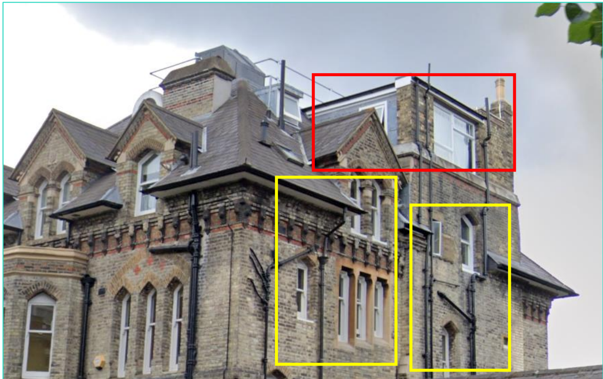
Site Facing Elevation – Upper floor fenestration
