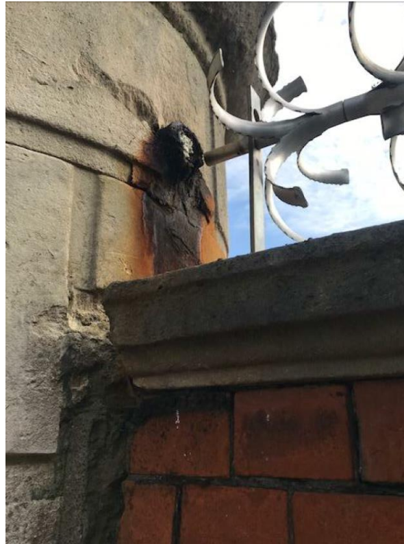
Figure 6 Southern pier of the pair to the west end of Mornington Street Railway Bridge, with evidence of former metal railings penetrating from the top of the stone piers
