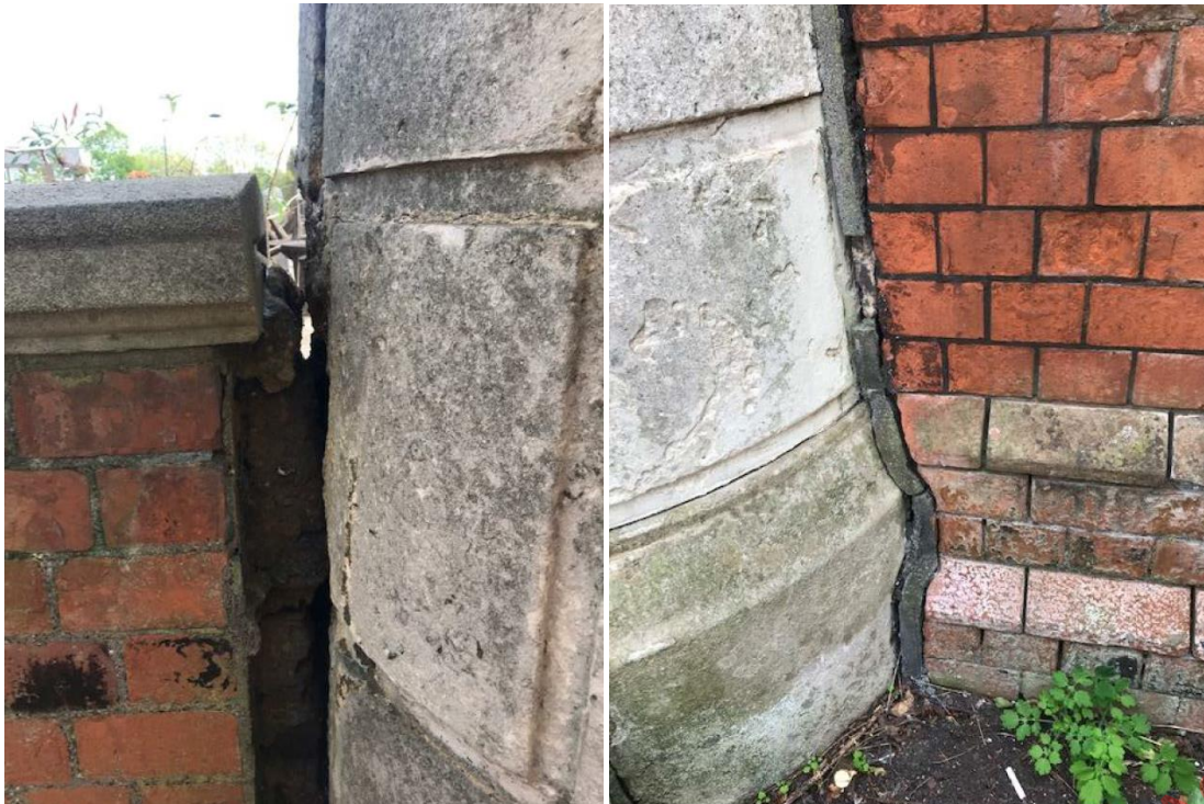
Figure 7 Northern pier (left) and southern pier (right) of the pair to the west end of Mornington Street Railway Bridge, with evidence of mortar packing between the stone pier and Park Village East wall
