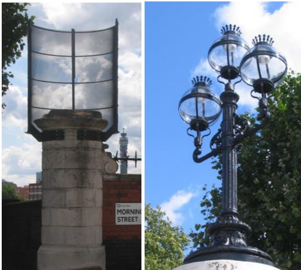
Figure 6 Images taken from the Cleghorn Lighting Ltd. website showing restoration works requiring the removal of the metal standard from the southern pier of the pair to the east of the bridge (left) and the standard and globes following works (right)
