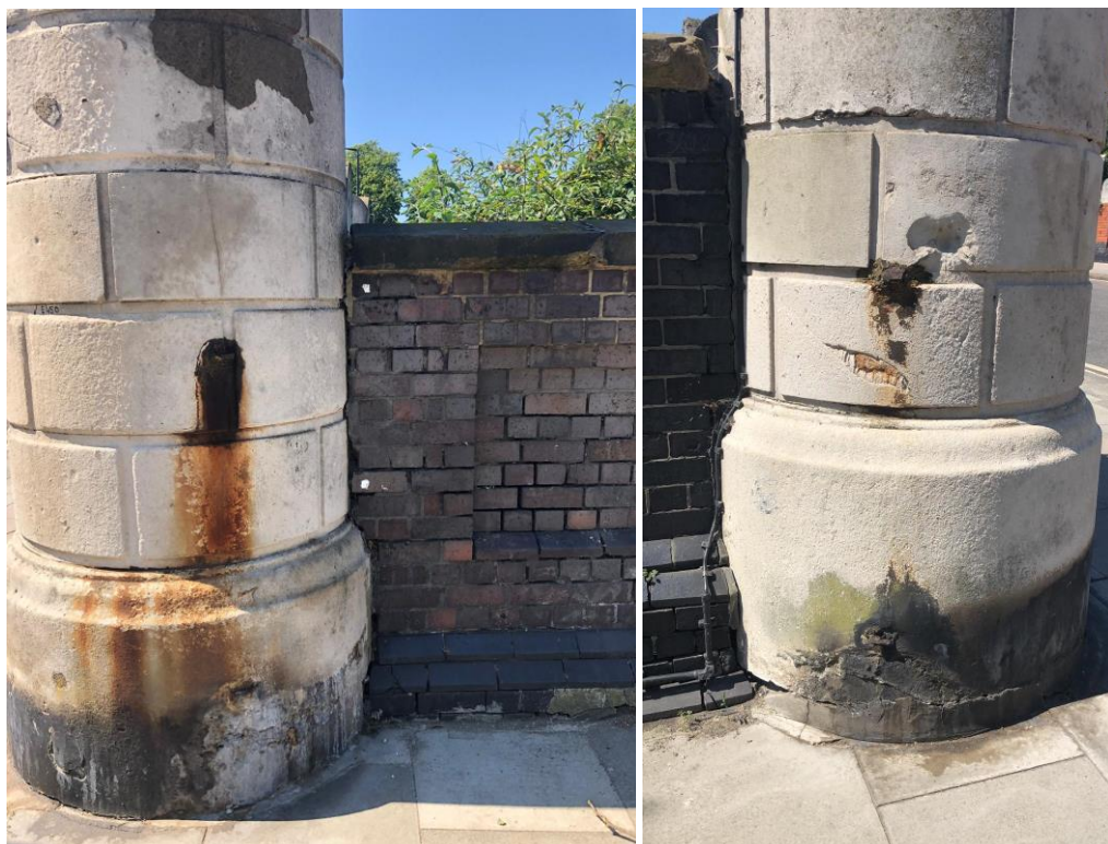
Figure 5 Northern pier (left) and southern pier (right) of the pair to the east end of Mornington Street Railway Bridge, with evidence of former metal work penetrating from the stone piers
