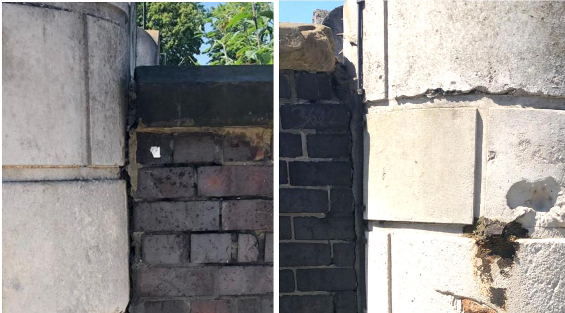
Figure 7 Northern pier (left) and southern pier (right) of the pair to the east end of Mornington Street Railway Bridge, with evidence of mortar packing between the stone piers and Mornington Terrace wall
