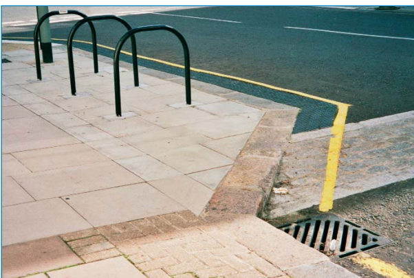
Footway build-out with cycle stands in Grafton Terrace
