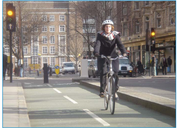
Segregated cycle lane in Torrington Place
