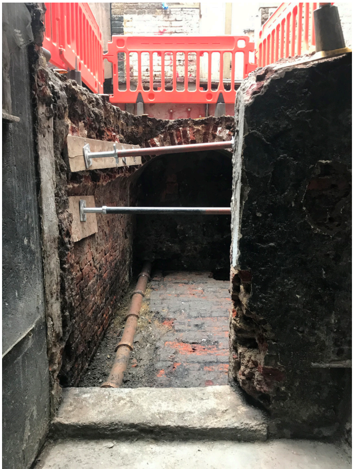
Vault 01 as seen from existing lightwell - lid of failed arch taken down and vault propped, ready for re-instatement
