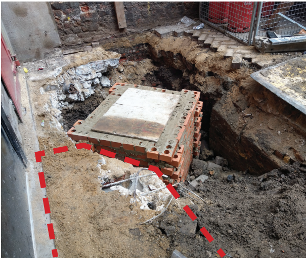
Existing coaldrop structure shown highlighted during drainage diversion works
