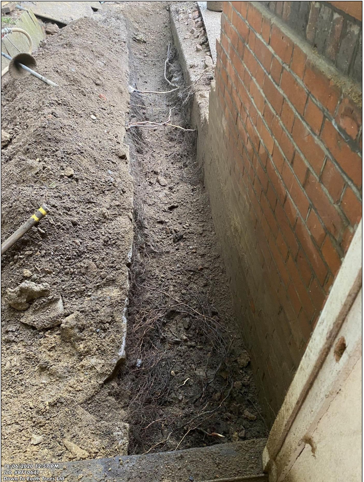
Photograph C – Showing fibrous roots adjacent to the existing building and 3 no. roots below 25 mm diameter which are outside the area of the proposed lightwell.
