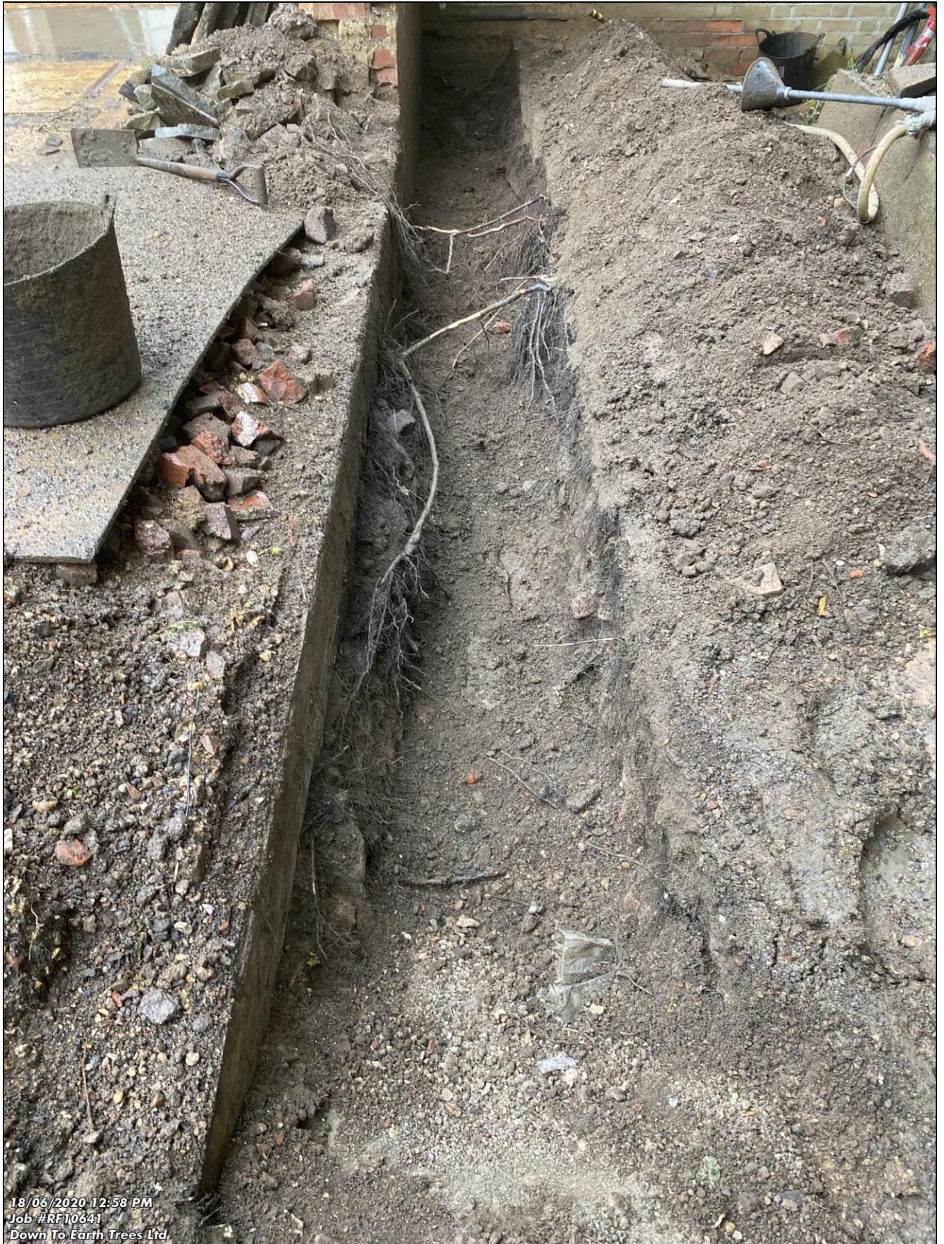
Photograph B – Showing the excavated trench.
