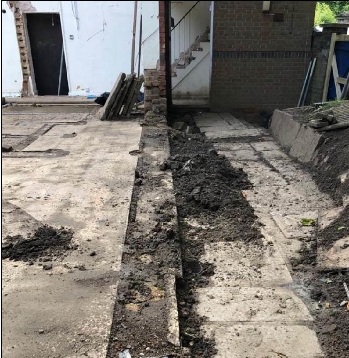
Photograph D – Showing trial trench being backfilled at the end of the investigations.
