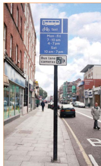
Separated signs carefully aligned on a post
