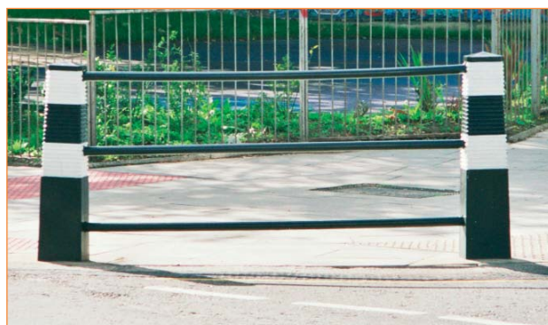
Bollards with railings
