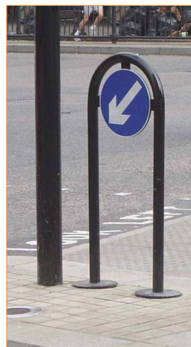
Externally illuminated metal hoop ‘keep left’ sign
