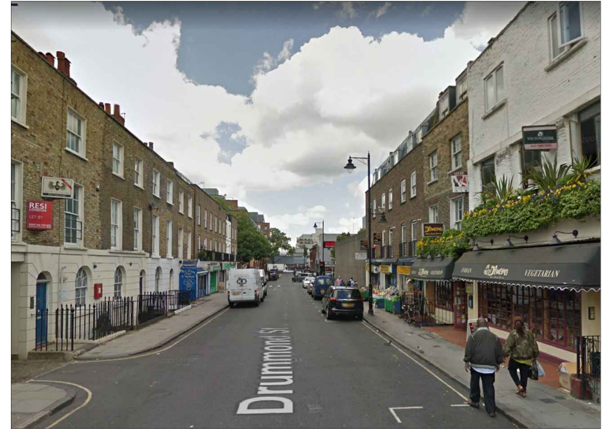
3 Existing Street View
