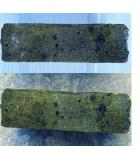
Spec: Existing brick cleaned of all paint and lightly sootwashed Finish: Sootwashed, level of sootwash to be confirmed by LPA
