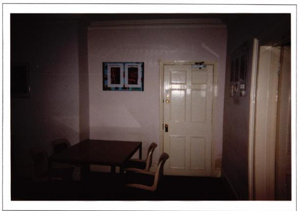
Photograph of the existing door to be removed and the opening to be infilled and the wall reinstated to it's original appearance. The door links the staircases to Nos 14 and 15 Southampton Place at second floor level. The photo is taken from the restroom to No 14 Southampton Place. The door opening is modern and was inserted within the last 10 years.
