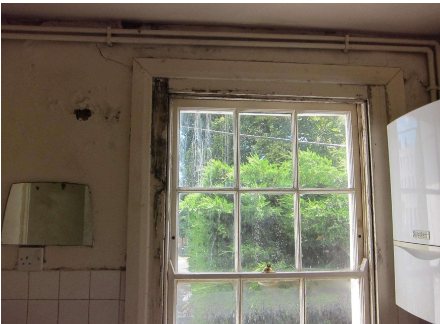
Water damage around kitchen window
