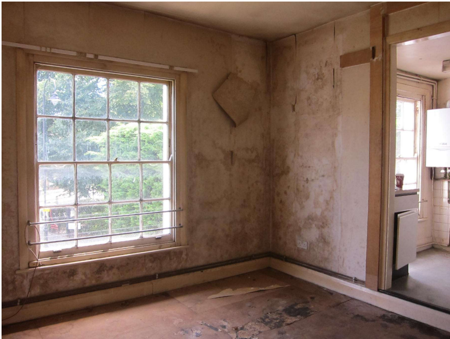
Living room showing water damage to front elevation and damage to flooring
