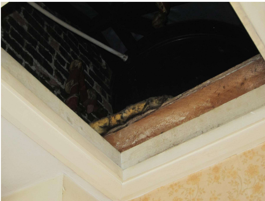
Ceiling hatch showing insulation
