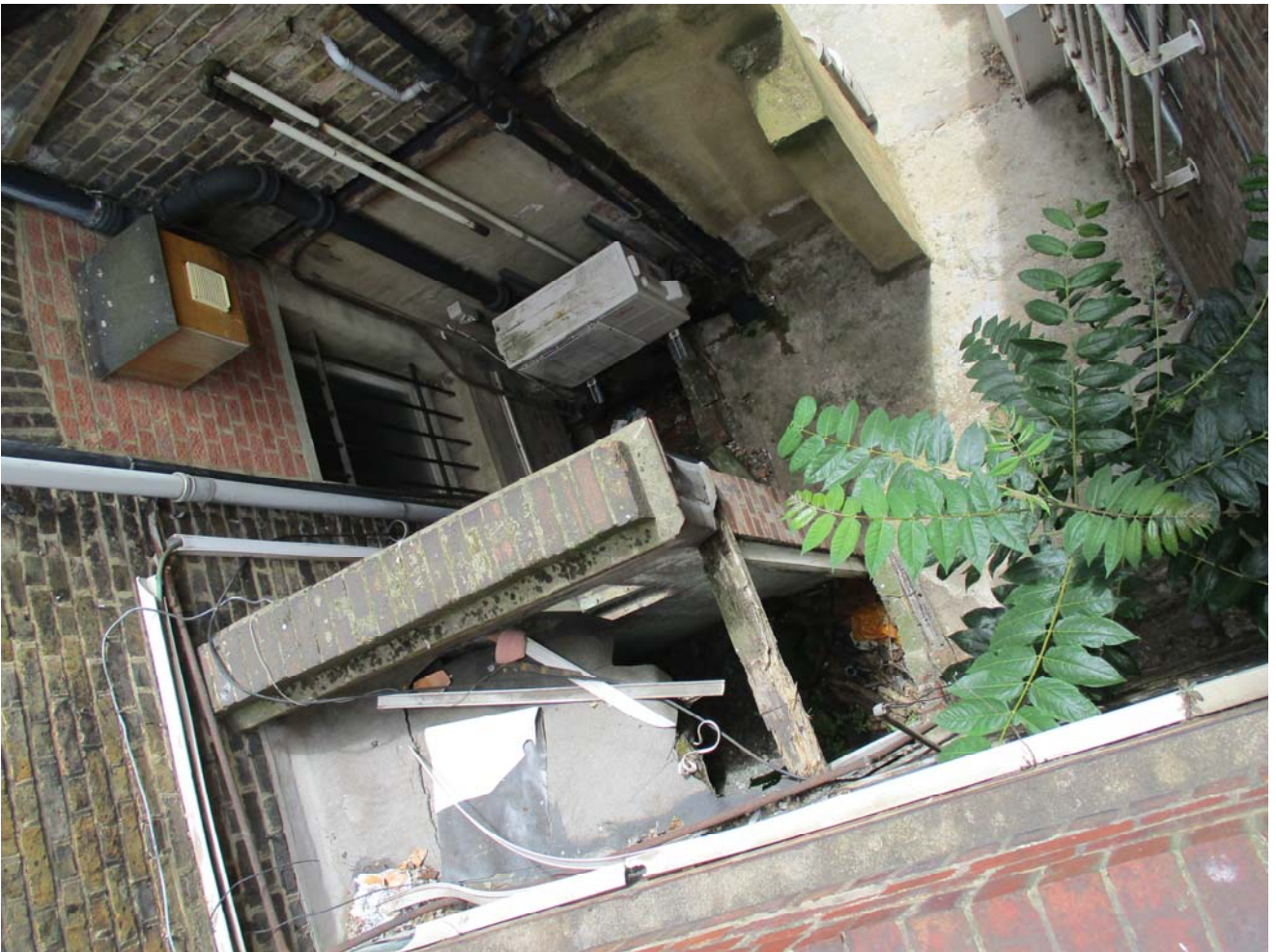
VIEWS OF REAR LIGHTWELL AT 105 CAMDEN HIGH STREET
