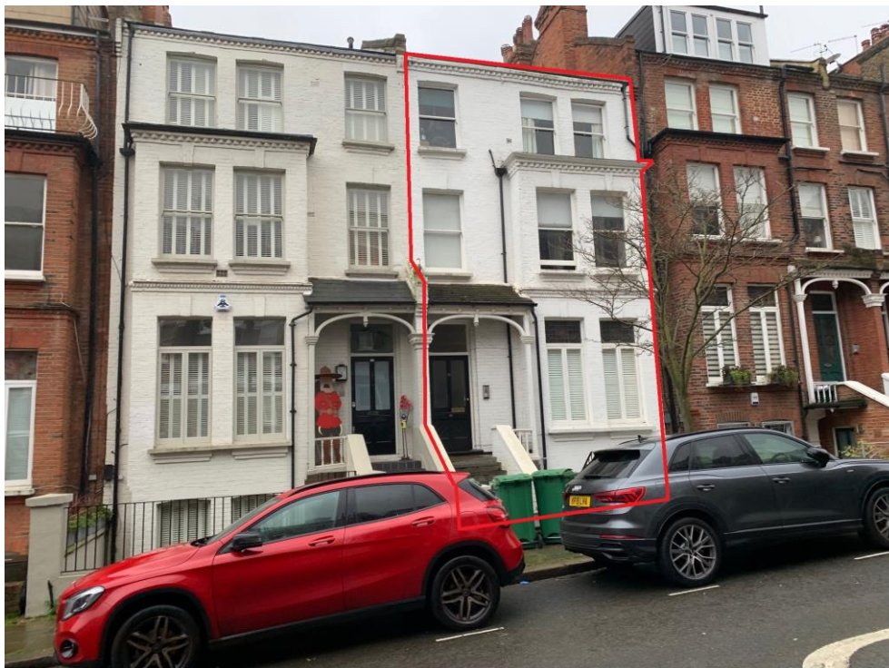
Application property, front elevation.
