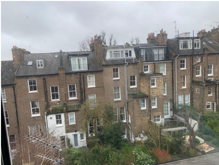
View of the rear rooflines of Kemplay Road properties facing Carlingford Road. The photograph was taken looking out of the existing dormer window of the application property.
