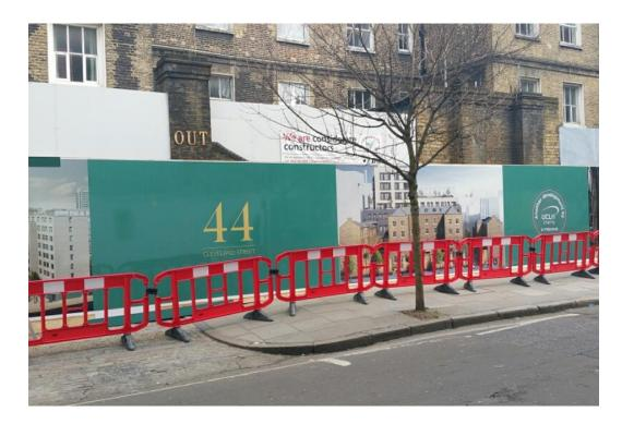
A site hoarding will be installed to the front elevation on Tottenham mews and anti climb Heras fencing to the north elevation between the two construction sites, further Heras to be applied to the upper scaffold lift preventing access from the adjacent site on the south end of the site also to where the scaffold is close to the Middlesex House external fire escape stair.
