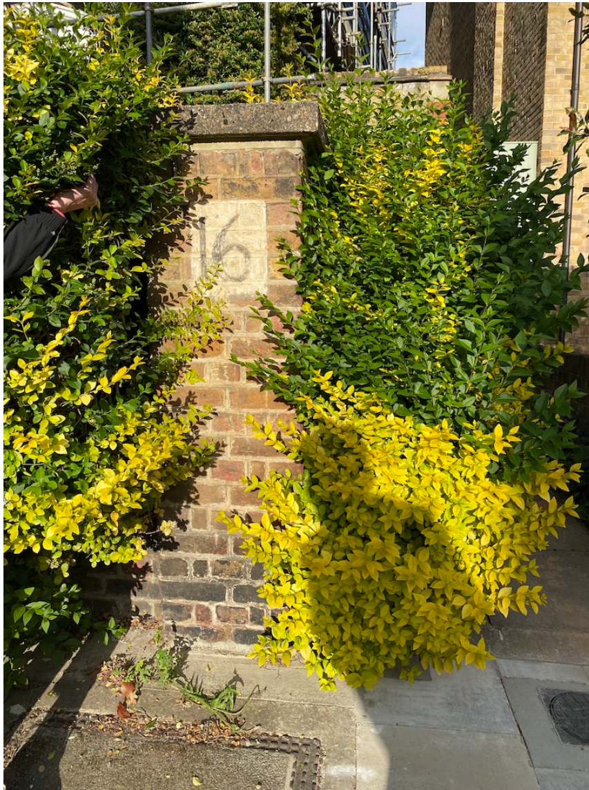
Right hand side pier
