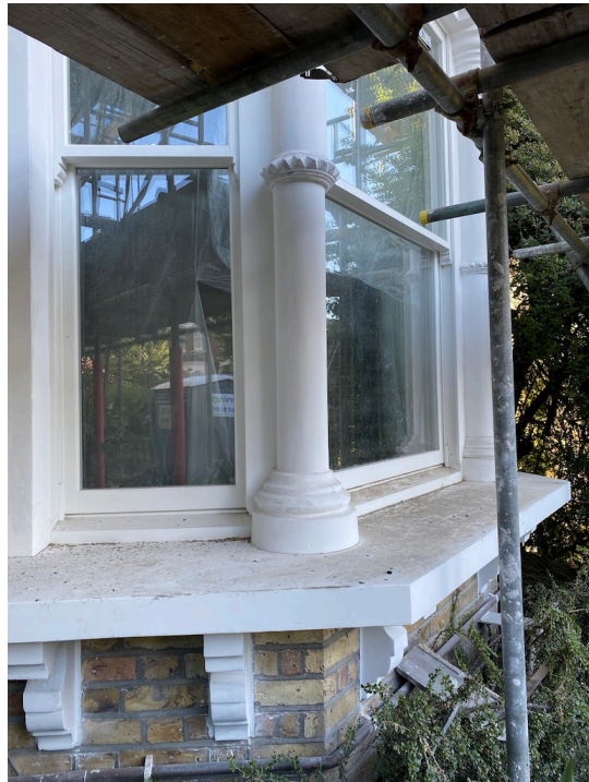
External renovations in progress
