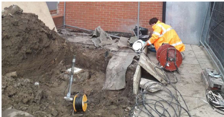
Plate 2: Seismic data collection setup at BH2
