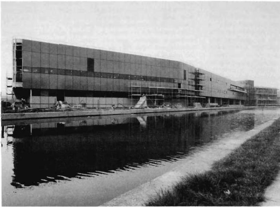
Fig 11. Canal elevation cladding nearing completion
