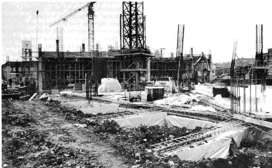
Fig 9. Clayboard protection to ground beams
